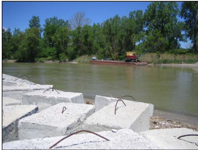
Figure 5. Erosion prevention measures along shoreline.
