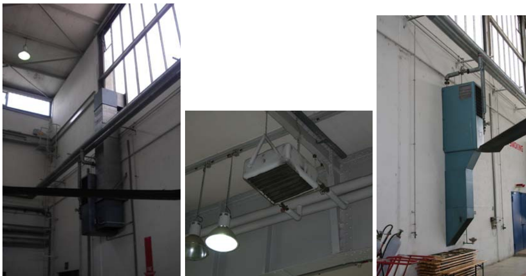
Figure 15. Typical warm air heating units used in hangars.
