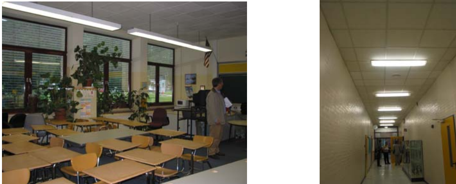
Figure 30. Suspended acoustic ceilings in classroom and traffic areas.
