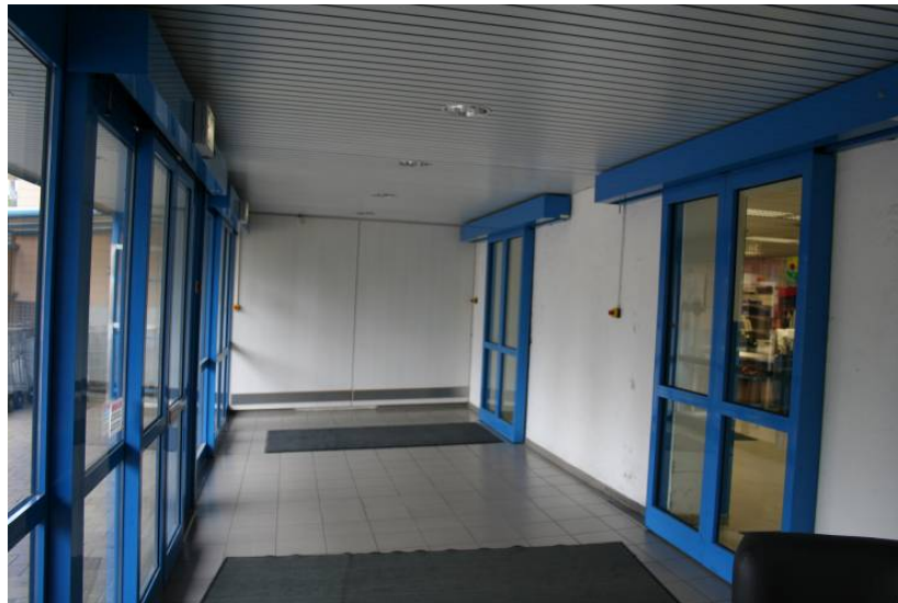
Figure 14. The Commissary at Katterbach, Building 5805.
