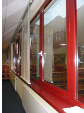
Figure 26. Double glazed red aluminum-framed windows.
