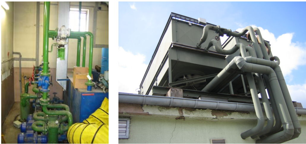
Figure 10. Cooling system pumps and cooling tower in Building 2362.
