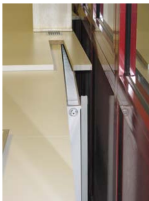
Figure 34. Elementary School cupboards placed in front of the convectors.
