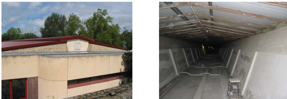
Figure 31. Second floor inclined roof.
