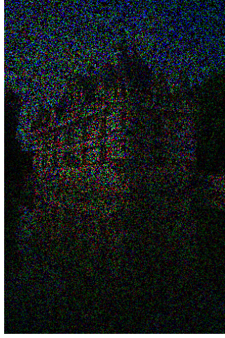
(b) Damaged Image
