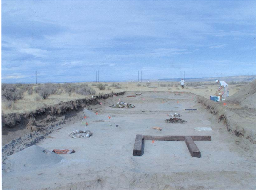
Figure 20: Construction of the Hammer test bed. In this sandy soil area mostly objects were laid in the ground and covered with homogeneous sandy silt.
