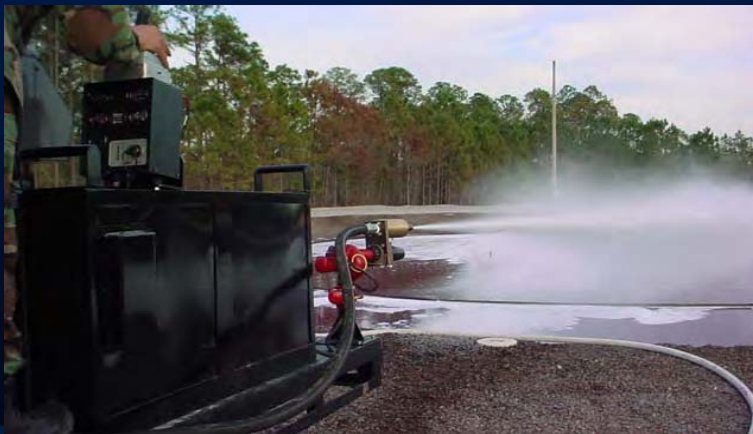
Apr 2004: 100 gpm UHP Skid
