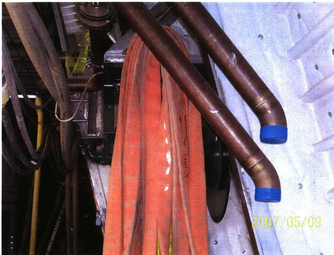
FIGURE 3. Starboard AFT AFFF Hose Reel Looking FWD. Note piping blocking hose payout.
