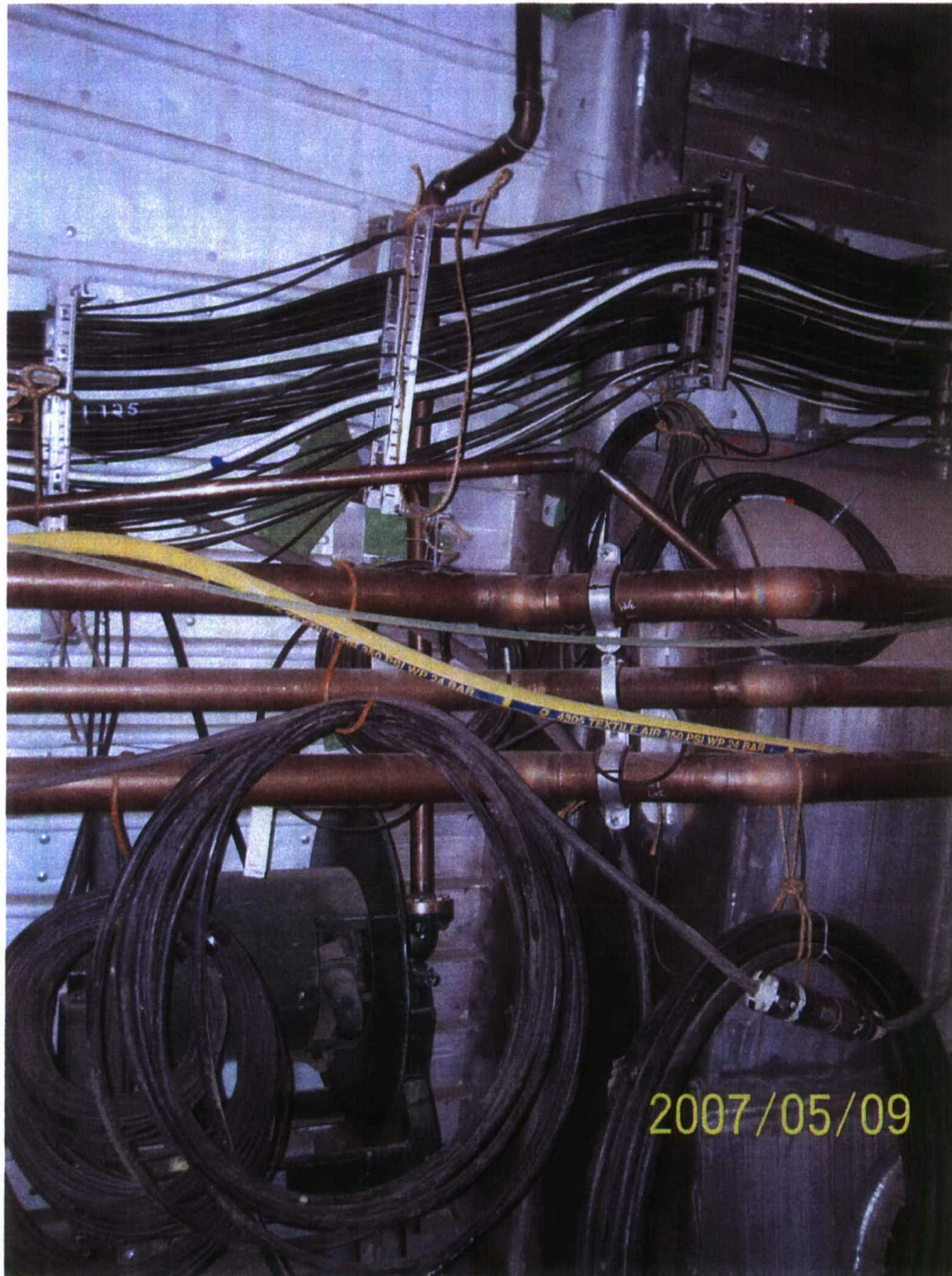
FIGURE 13. Lower Portion of 1-1/2" Piping Feeding STBD FWD Reel. Note number of bends in runs that will lead to a reduction in pressure at reel.
