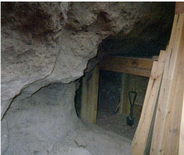
Figure 5. At the bottom of the shaft as the tunnel or adit is going into the unconsolidated – silt interface. Note the bedding plans outlined by stained grains in the unconsolidated sand layer.
