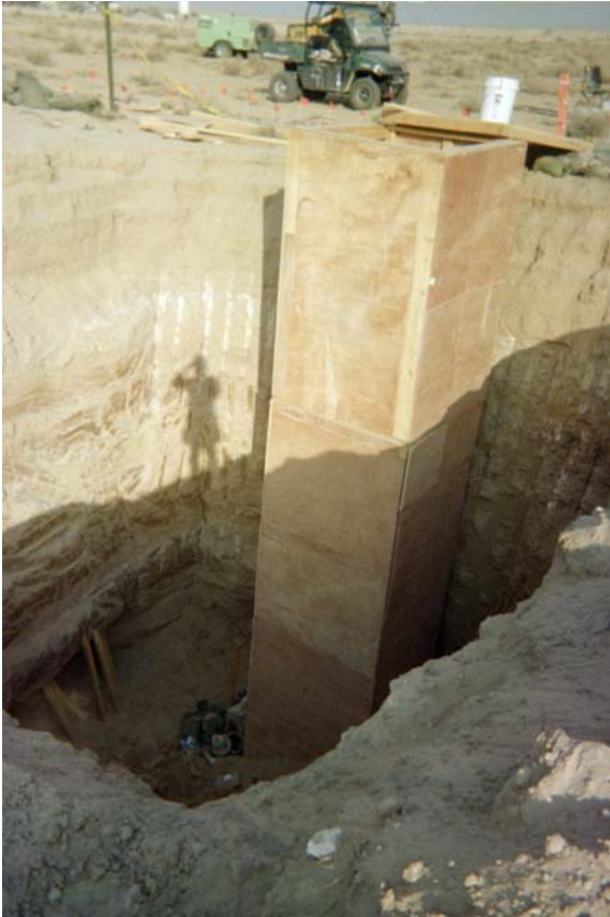
Figure 4. Shaft in place. Note the various layers.
