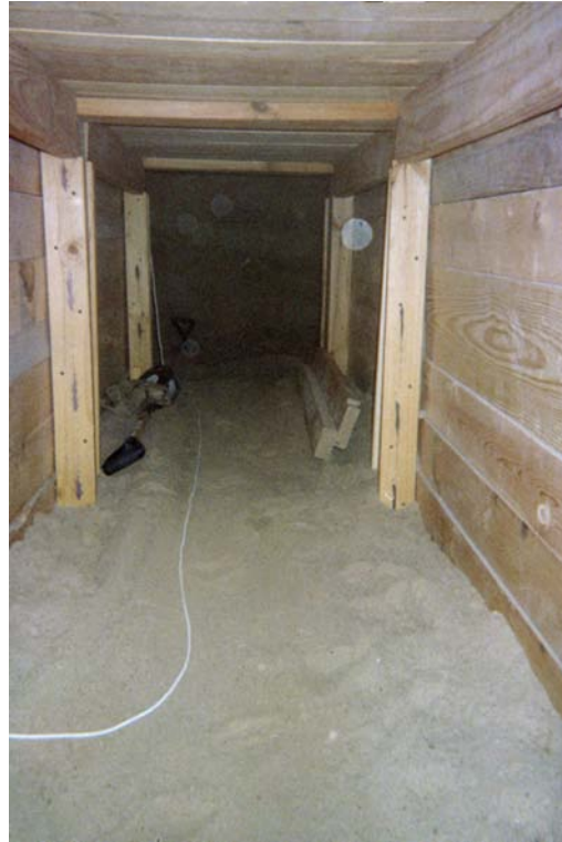
Figure 6. A look down the adit to the working face.
