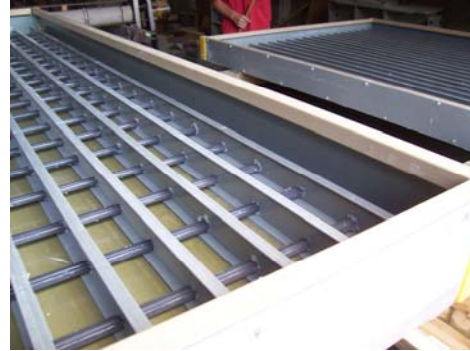
Fig. 8. Stay-In-Place Form and Reinforcement
