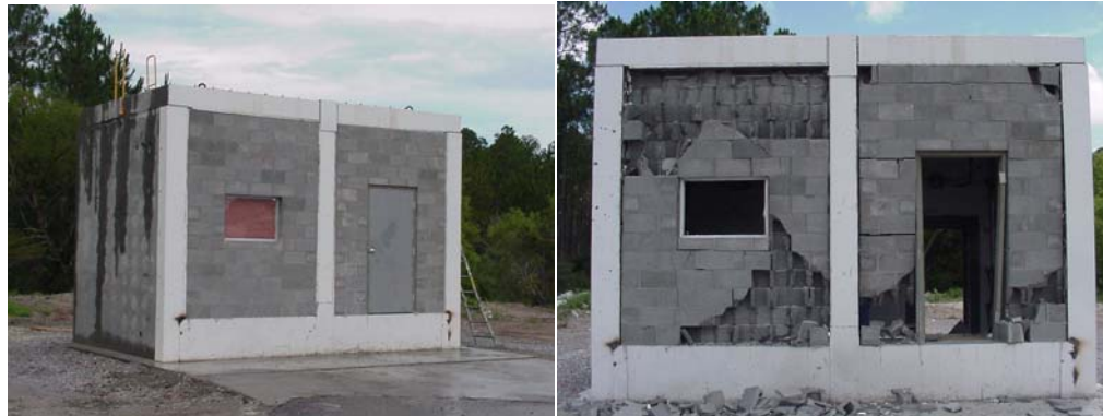
Fig. 3.1-6: Pre- and post-test pictures of walls in test 9
