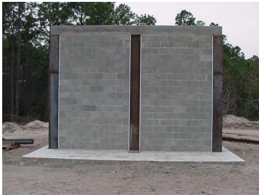
Fig. 3.1-2: Typical finished test walls
