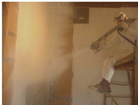
Fig. 2.3-1. Application of spray-on polymer
