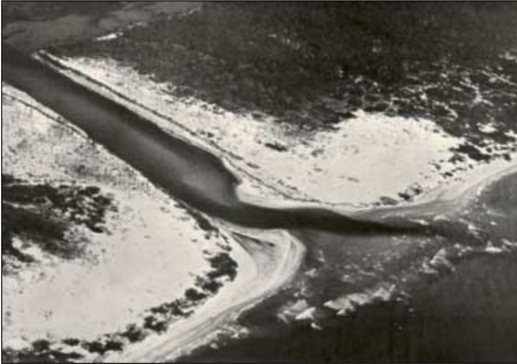
Figure 1. St. George Island Channel, Florida, before jetties (1955).
