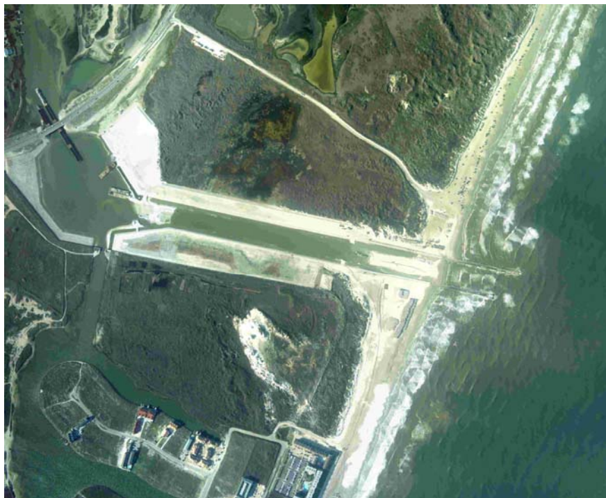
Fig. 2. Packery Channel (Inlet), Texas, under construction, March 2005
