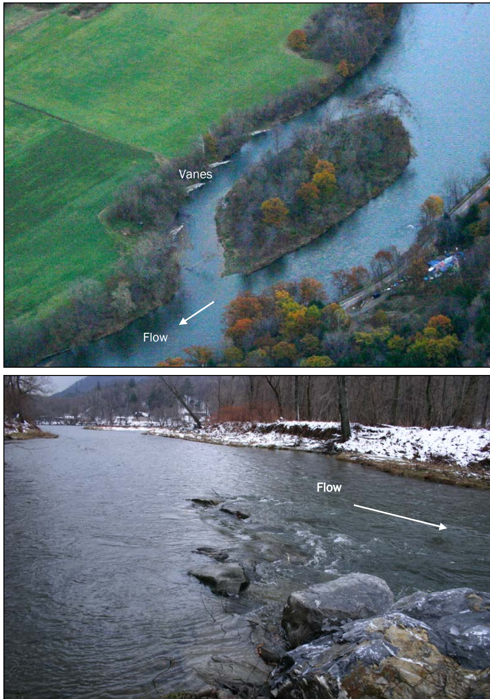
Figure 1. Rock vanes designed by NRCS to stabilize bank of the Winooski River at Bolton, Vermont.
