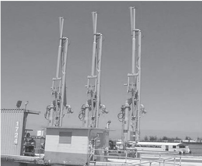
A refueling pier critical to sealift port operations.
