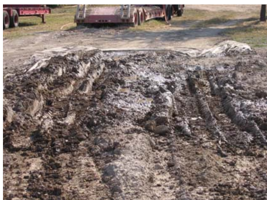
Figure 2. Constructed muddy driving area.
