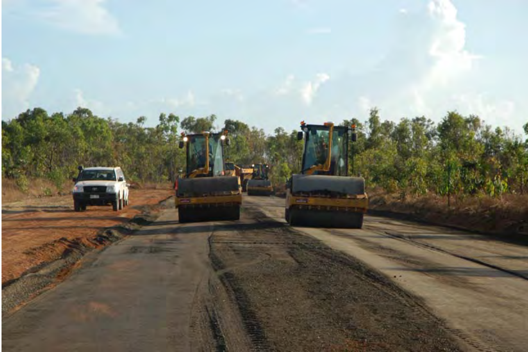
Figure 44. Compaction operations on the final lift during the MRX.
