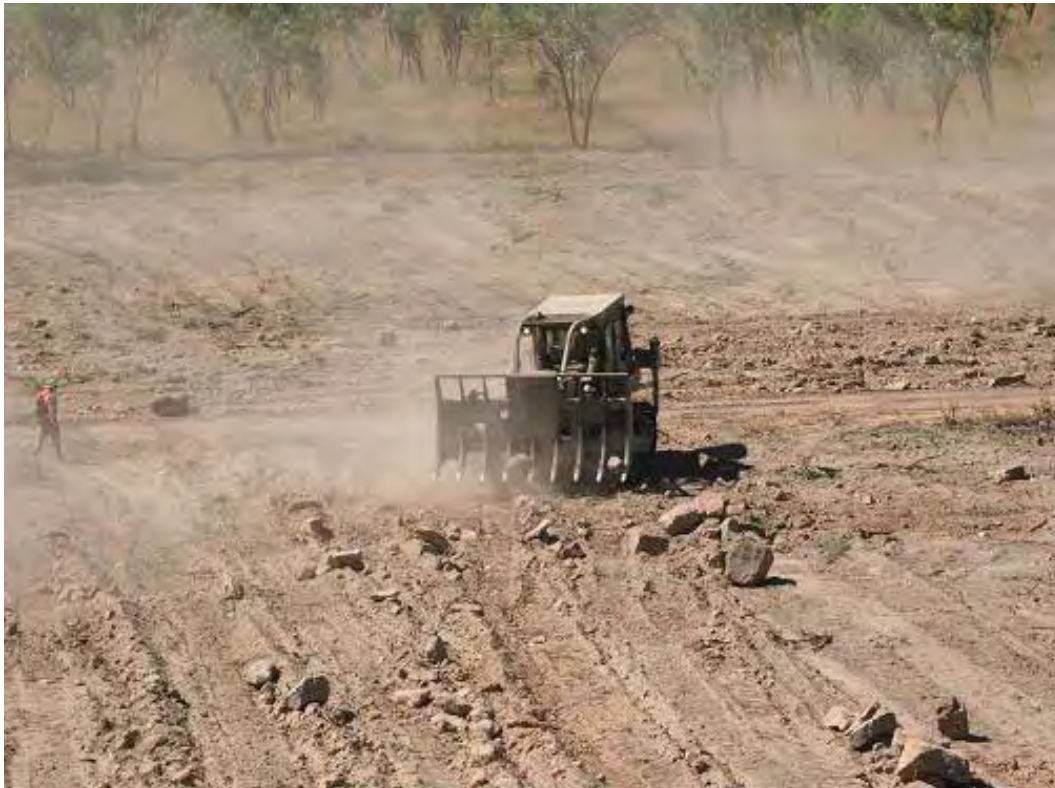
Figure 59. Komatsu D155 dozer clearing boulders in the subgrade layer.
