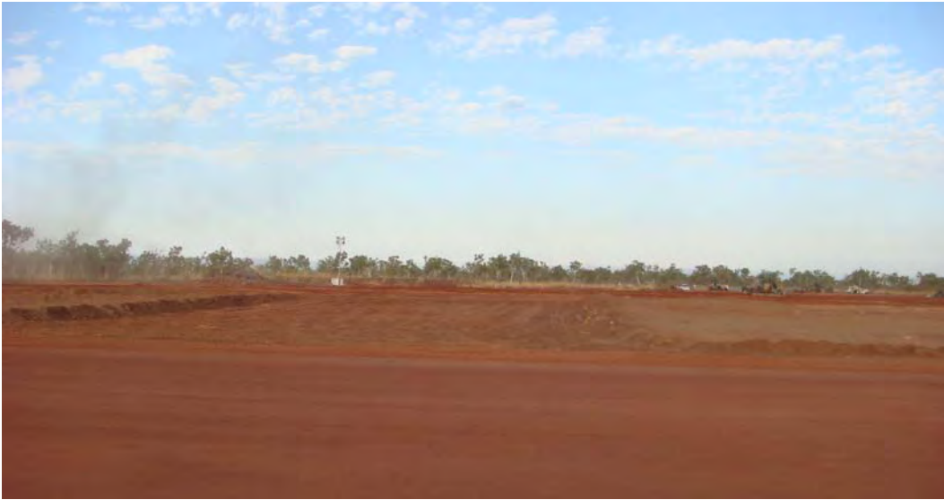
Figure 72. Box out of Taxiway Alpha prior to first rain event (18 June).
