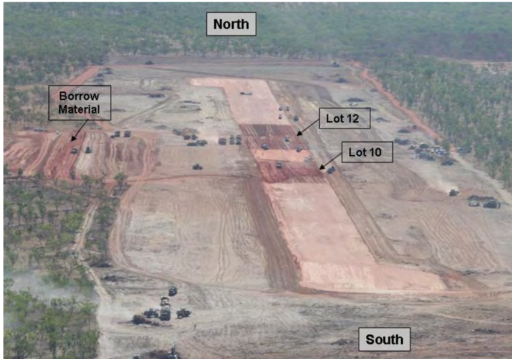
Figure 61. Completed base course and beginning of wearing surface construction on 12 June.
