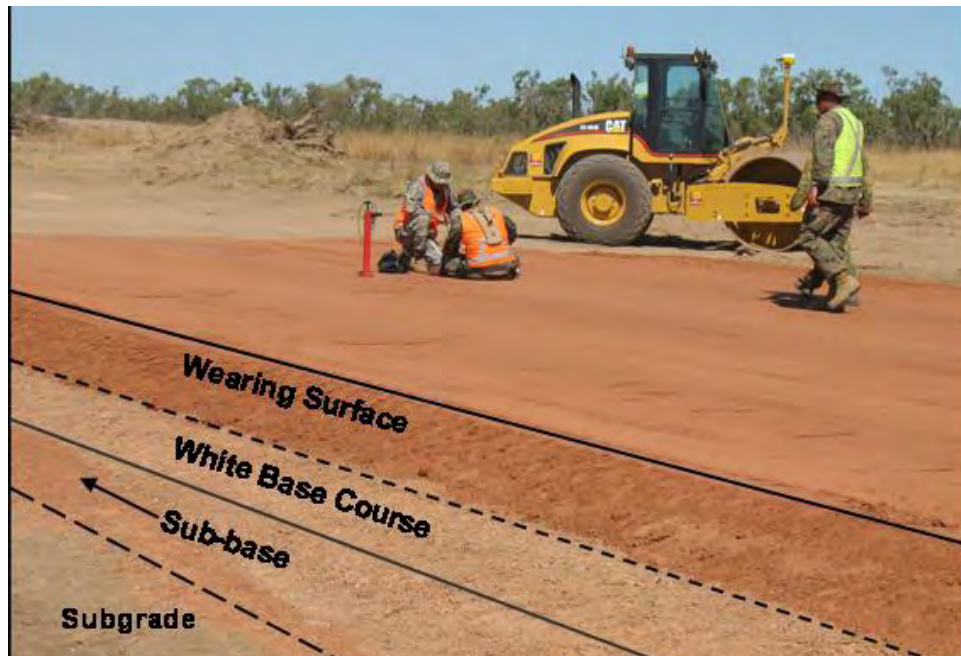
Figure 51. Layer construction of test strip.
