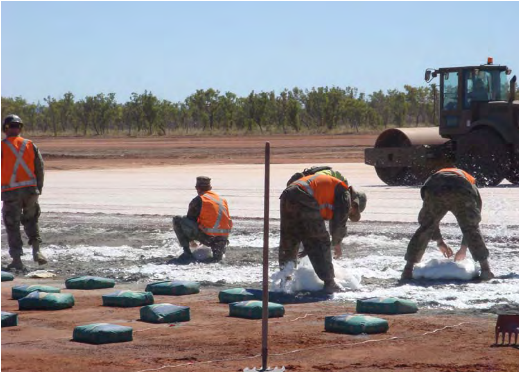
Figure 80. Placement of stabilizer materials on Apron Alpha.
