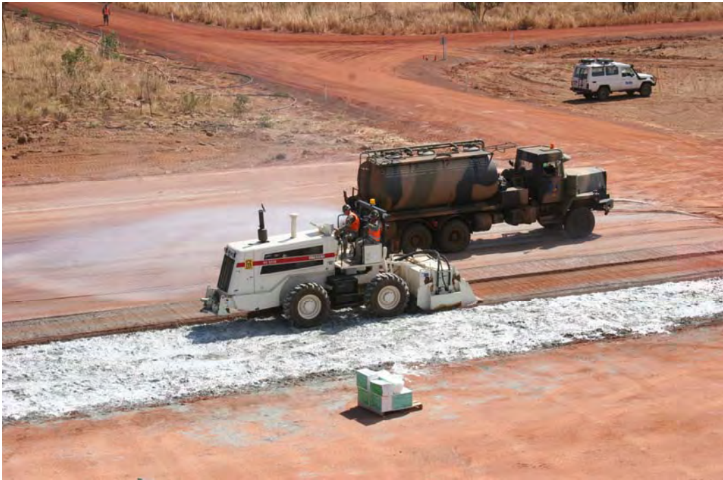
Figure 79. Stabilization training and construction of helipad.
