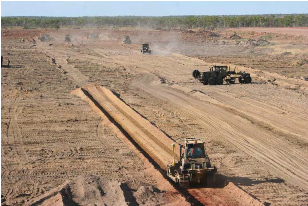
Figure 57. Boxing out of the subgrade.
