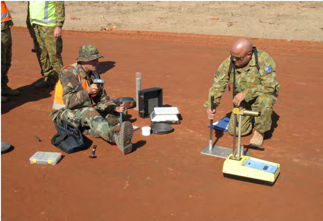
Figure 56. Steel shot replacement and nuclear gauge testing on the test strip.
