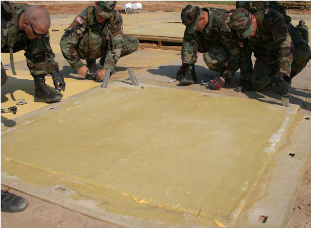
Figure 32. Placement of ACE matting.
