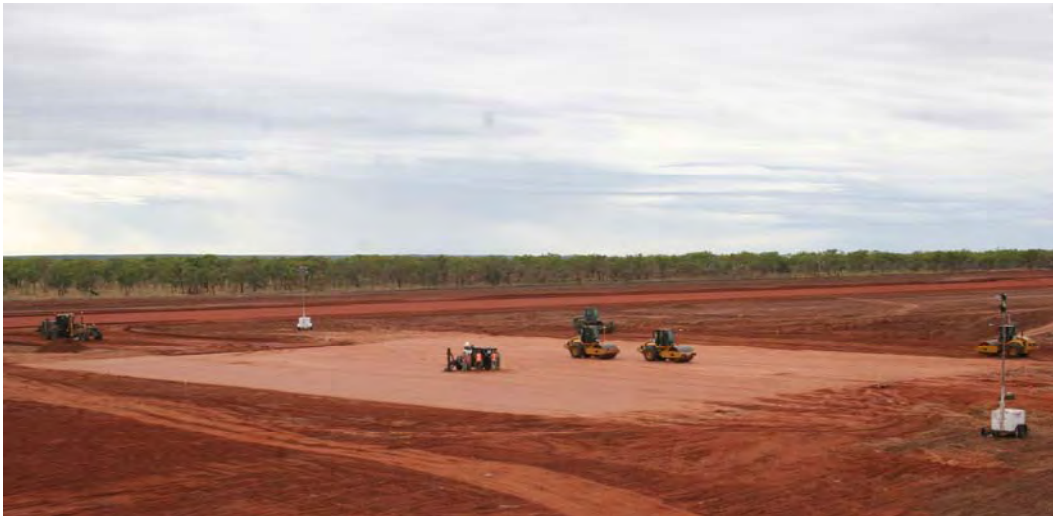
Figure 75. Compaction of base surface on Apron Alpha (24 June).
