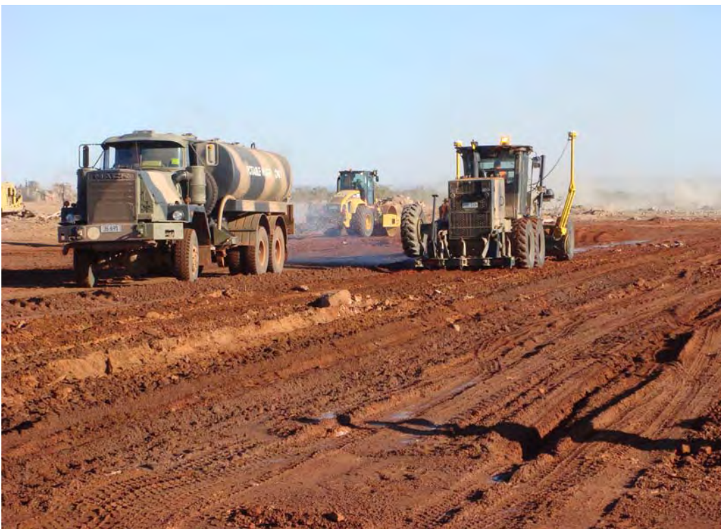
Figure 58. Subgrade and subbase preparation (7 June).
