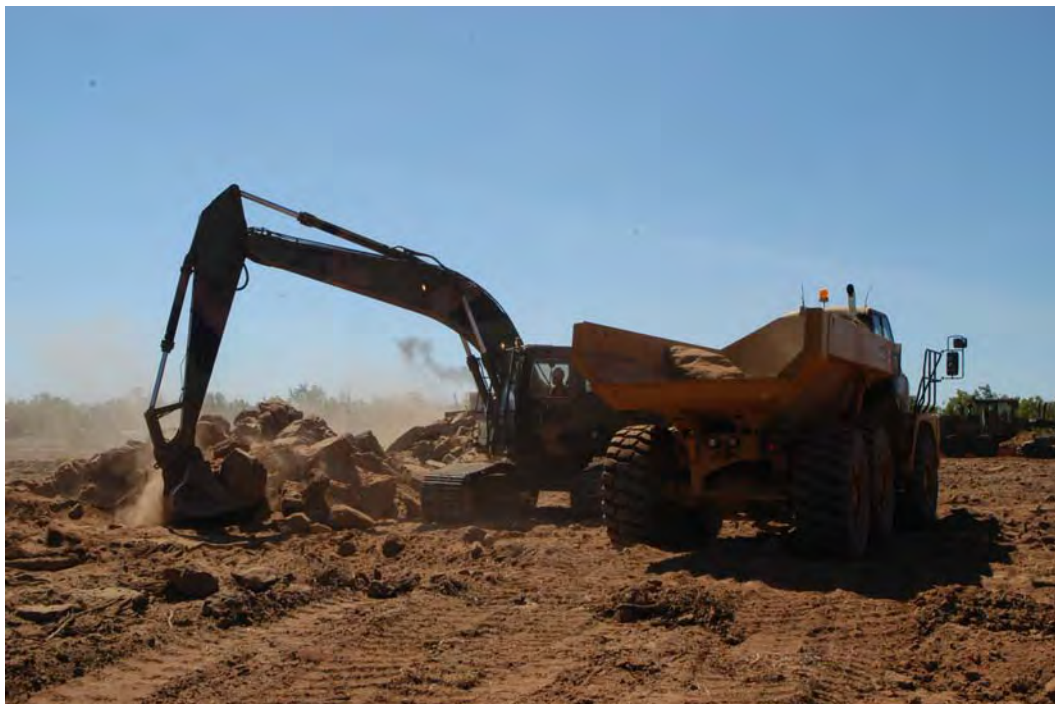
Figure 60. Handling of on-site boulders.
