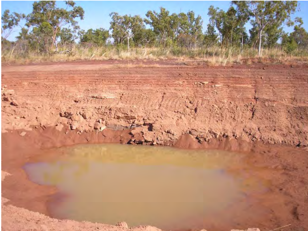
Figure 5. Example of a borrow pit used to obtain prepositioned material at BFTA site.
