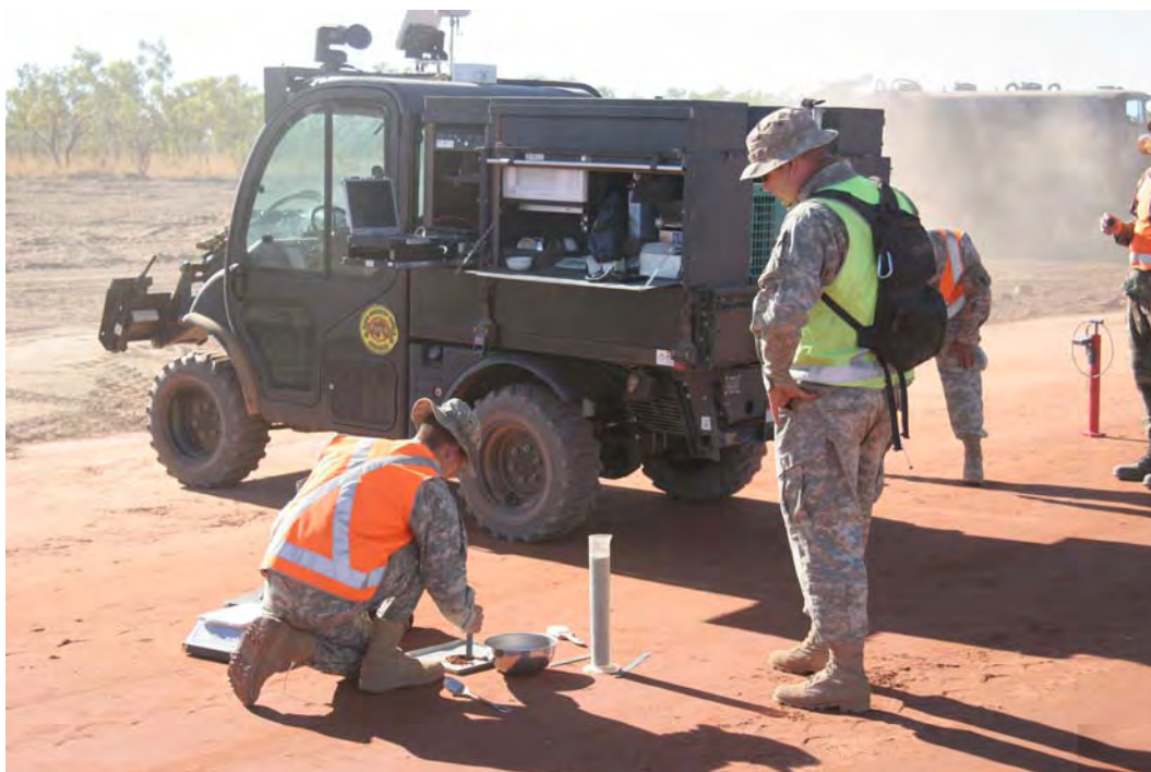
Figure 67. Steel shot density and Clegg hammer quality control on runway.
