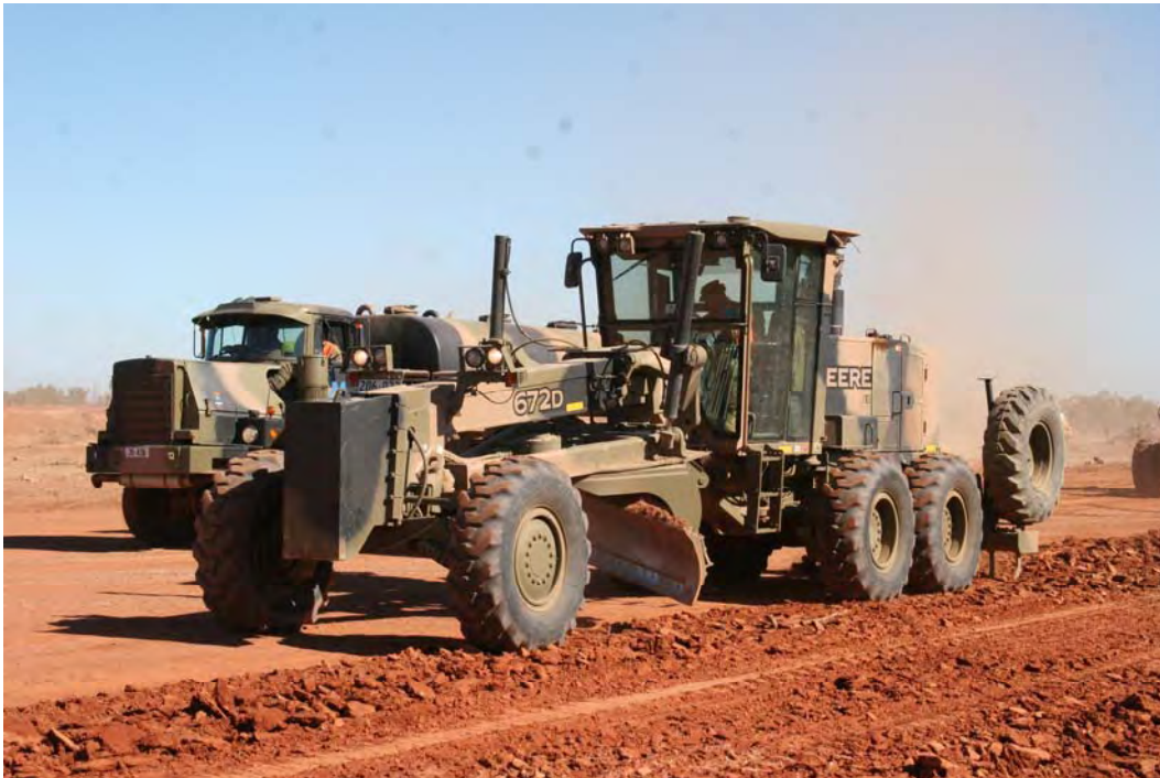
Figure 62. Scarifying base layer prior to placement of wearing surface.
