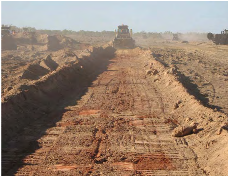
Figure 52. Illustration of test strip subgrade box out.
