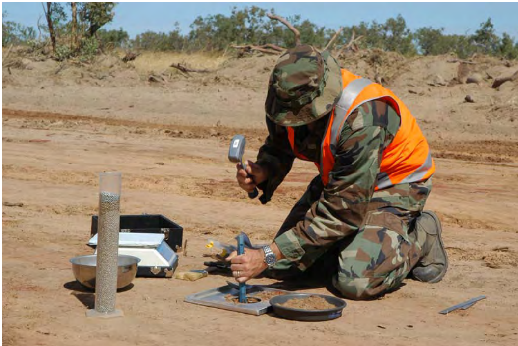
Figure 66. Soldier performing steel shot density test on improved subgrade soil.
