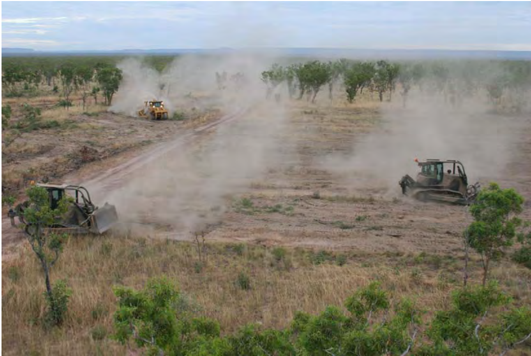
Figure 45. Clearing and grubbing of primary runway.
