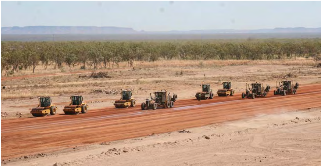
Figure 63. Compactor train during base course construction.
