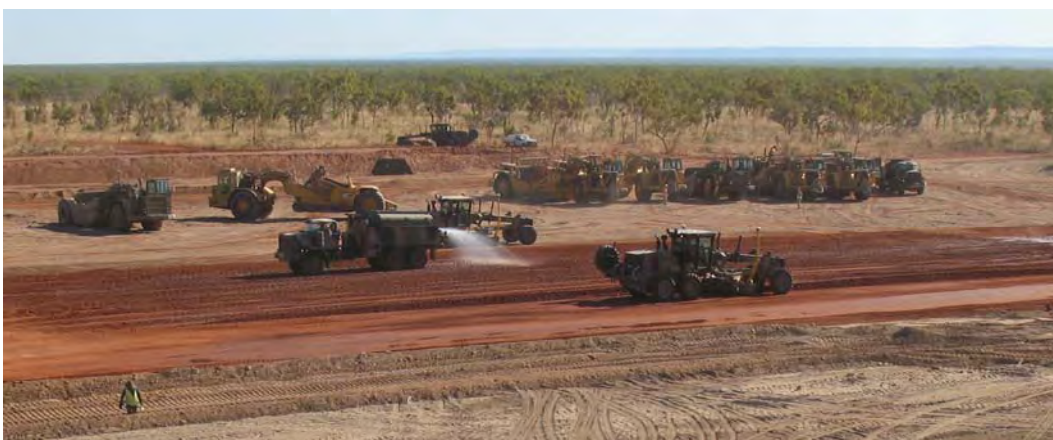
Figure 64. Water distribution on wearing surface while the grader blends in the water. CAT scrapers (yellow) and Komatsu scrapers (green) in background.
