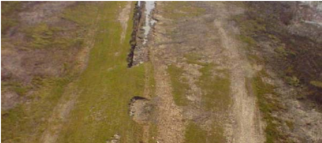
Figure 2. Crown erosion along MRGO levee in St. Bernard Parish.
