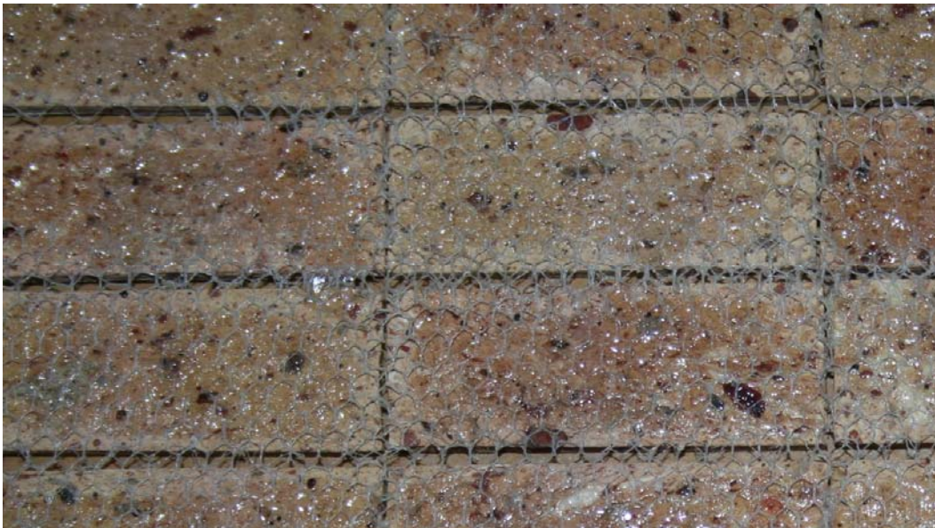
Figure 21. Mesh glued to underside of block mattress.
