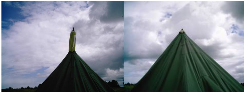
Figure 14. Tent peak damage and funnel repair at Ft. Lewis, WA site.
