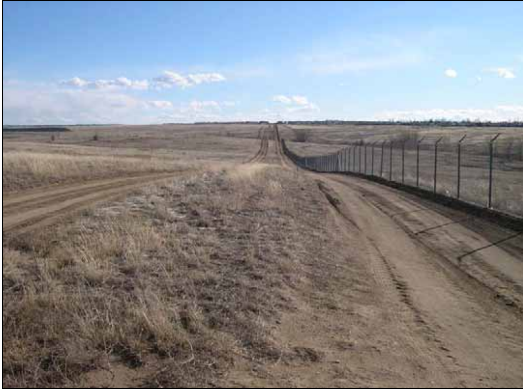
Figure 2-2. Split in the Perimeter Road
