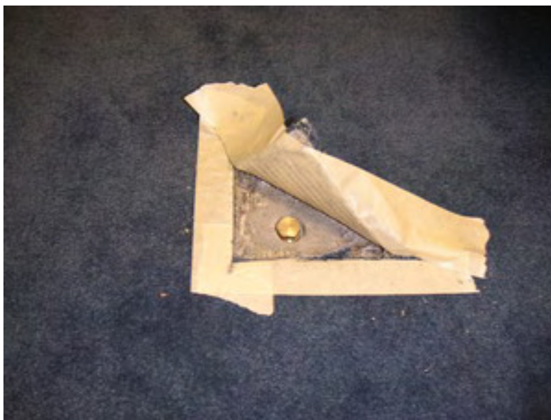
Figure 3.5.1.3 Sub-Slab Sample Port.
