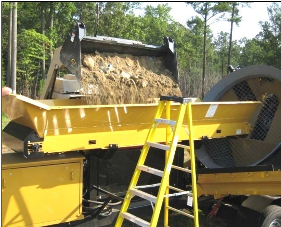
Figure 13: Material Loaded into Sifter's Hopper
