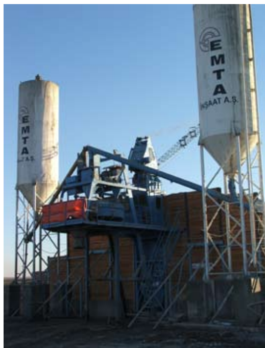
Concrete batch plant to mix concrete
