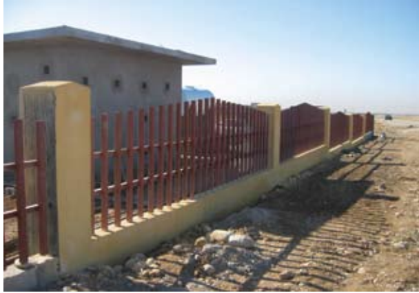
Perimeter fence segment.
