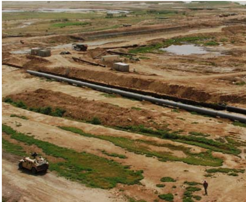
Welded pipe string at the Zegeton Canal
