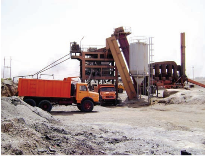
Renovated asphalt plant near Amara. (USACE photo)
