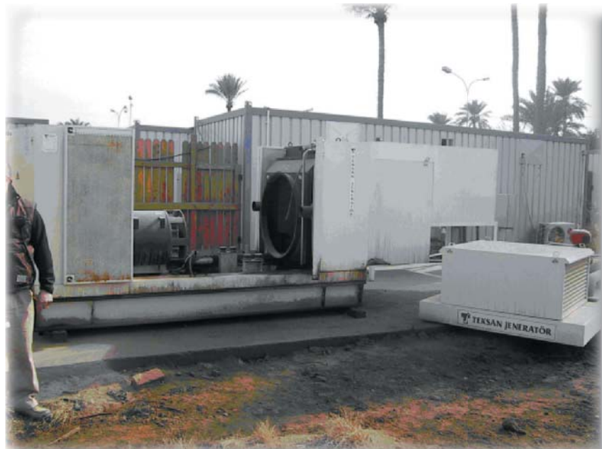
Shell for the 500-kilowatt generator undergoing repairs at the Babylon Police Academy.
