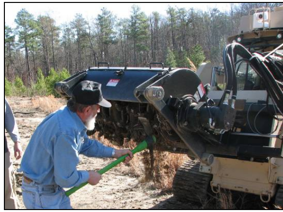
Figure 54: Removal of Dirt and Vegetation Accumulation
