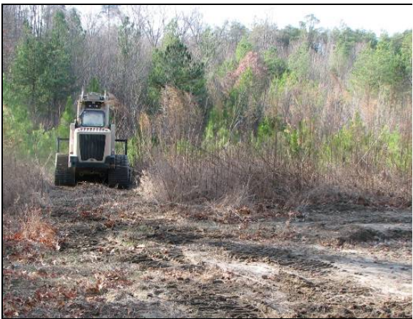
Figure 25: Category 1 Vegetation, Before Cutting
