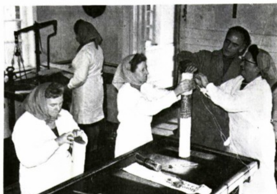
FIG. 6. 120 mm. L11 bag charges being made up Note the lead foil used as a de-coppering agent
