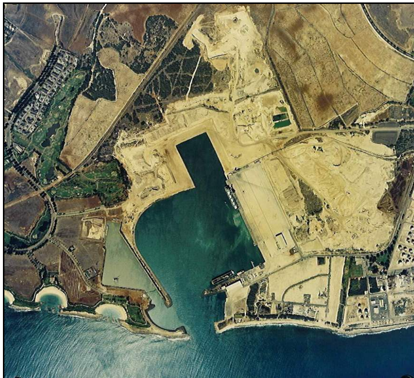
(b) Overhead view.
