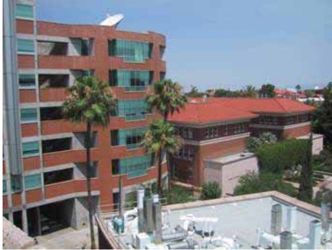
Figure 10. View from the roof of Shantz looking northwest.
