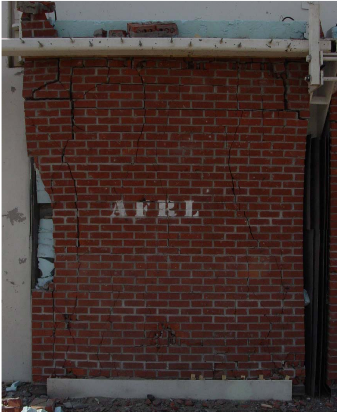
Fig. 3.49. Exterior view of Wall 2 after Detonation 3
