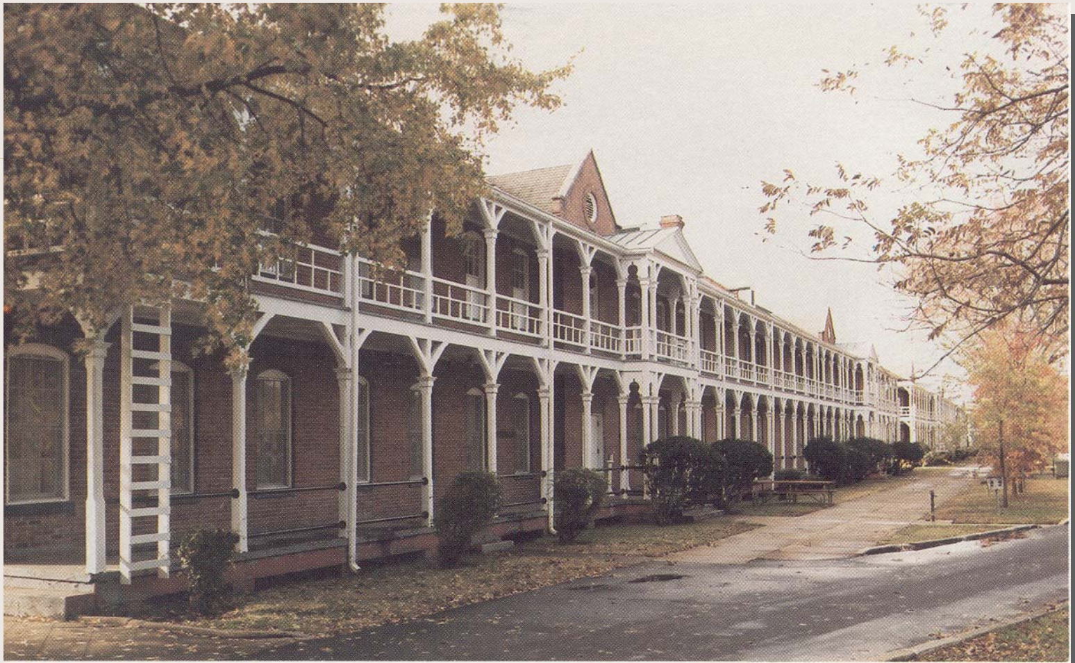
Figure 78. Troop Row Barracks (Bldg. 56), 1984
