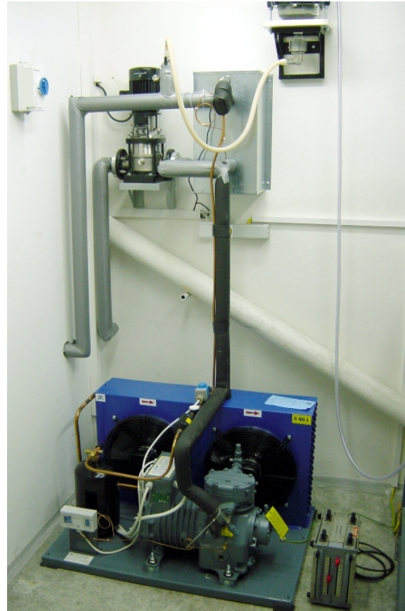
Photo 19. Cooling unit for ethanol cooling in trap
