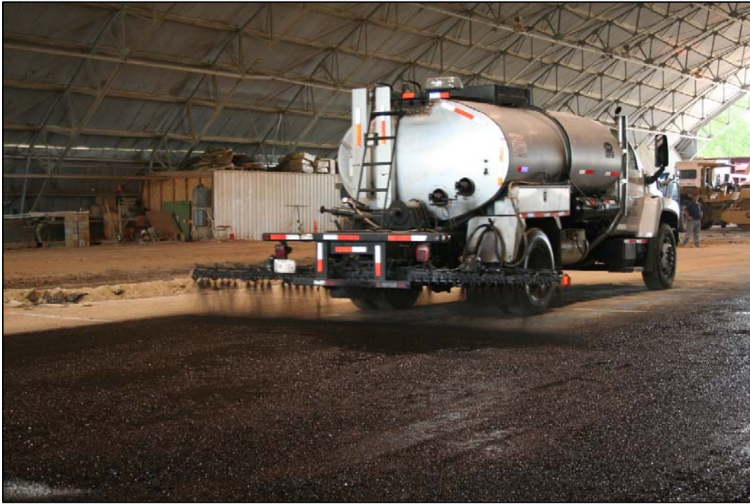
Figure 16. Applying the prime coat.
