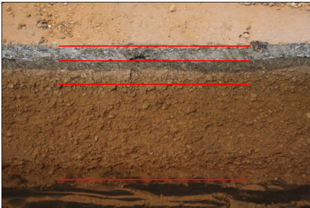
Figure 38. Item 1 trenched profile view.
