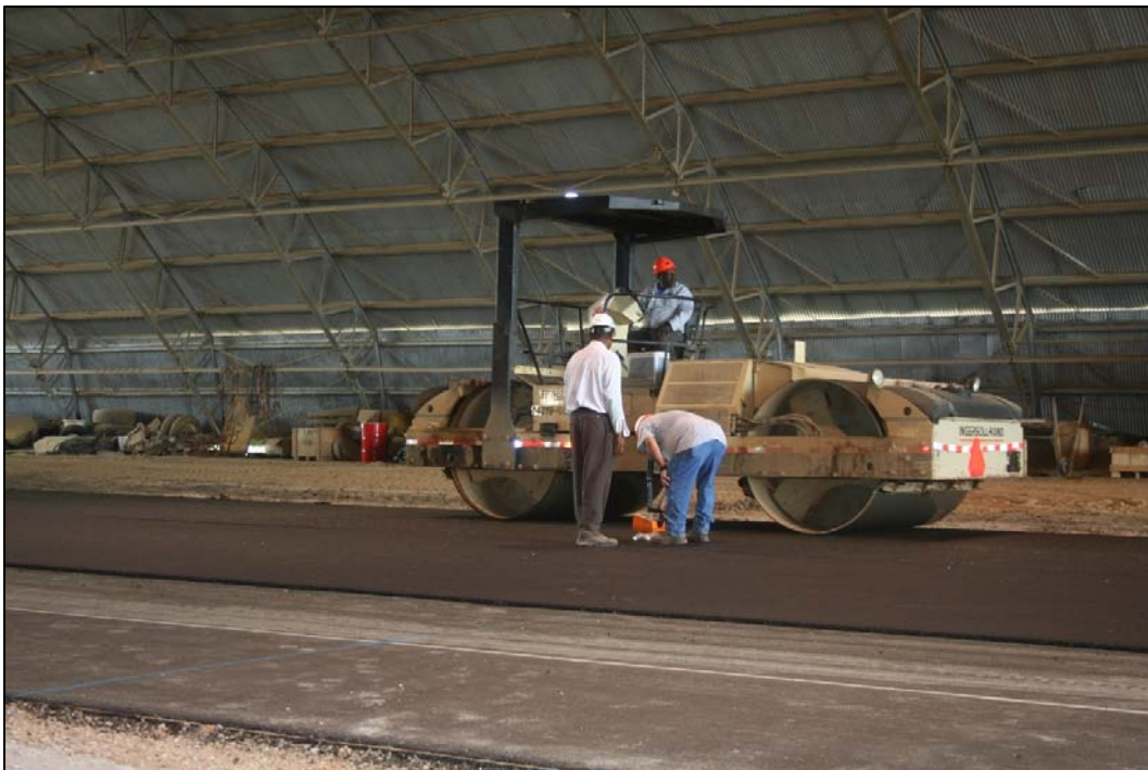
Figure 17. Compacting the asphalt concrete and taking density measurements.
