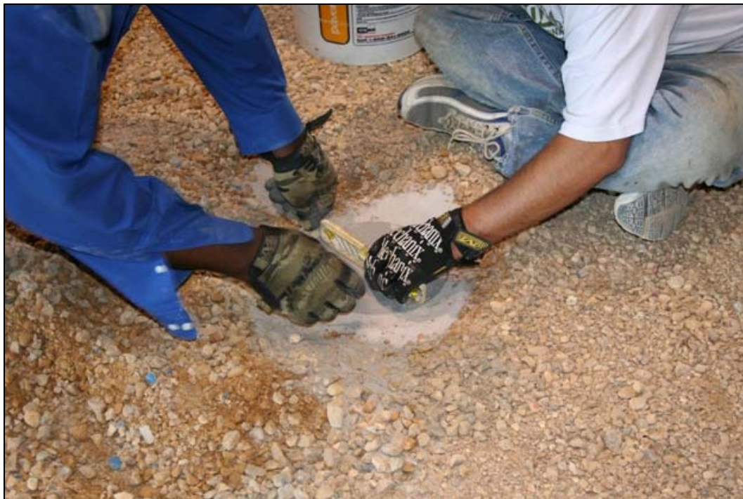
Figure 18. EPC installation in a crushed gravel base course layer.
