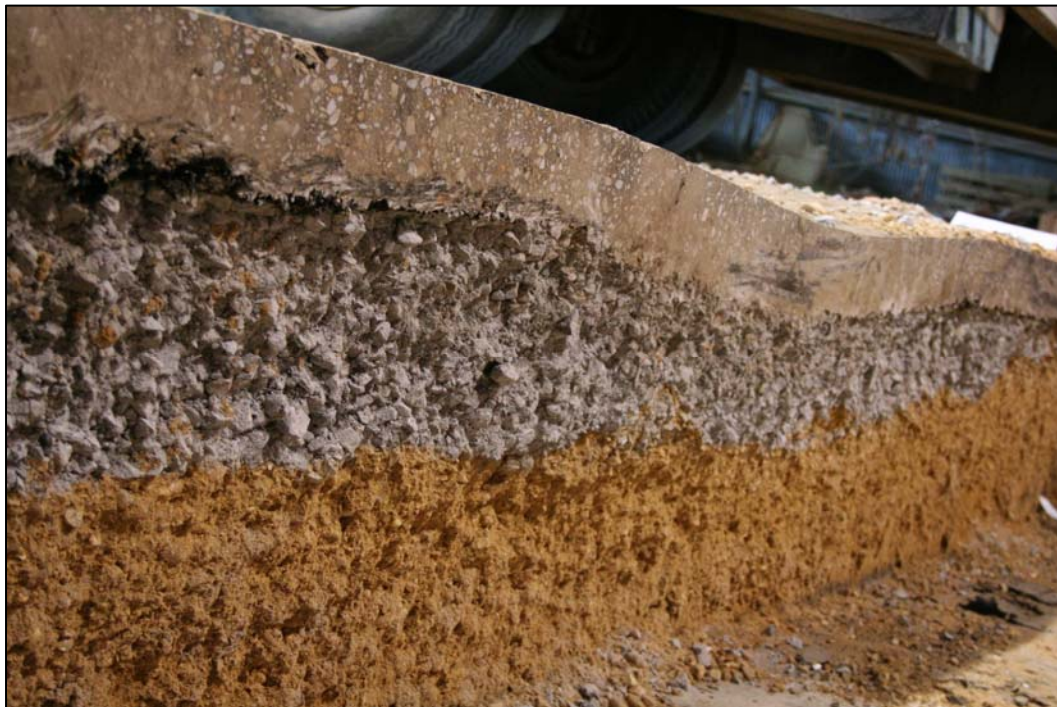
Figure 72. Item 4 trenched profile view.
