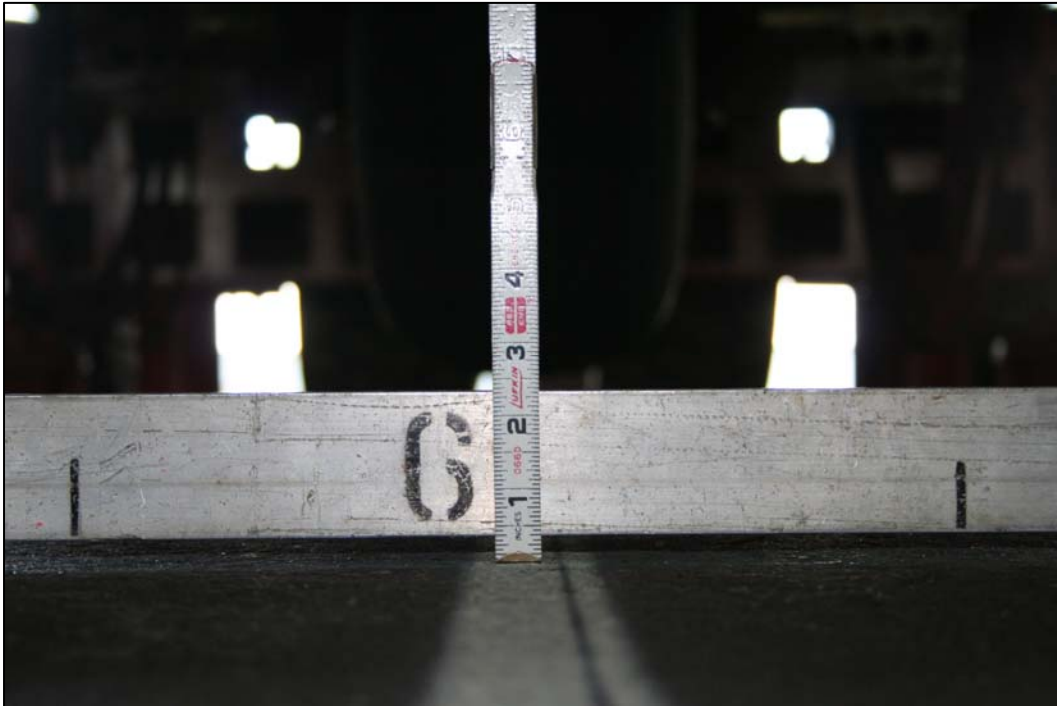
Figure 51. Item 3 rutting after 147 passes.
