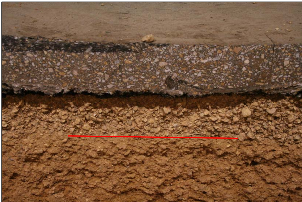
Figure 94. Item 6 trenched profile view.
