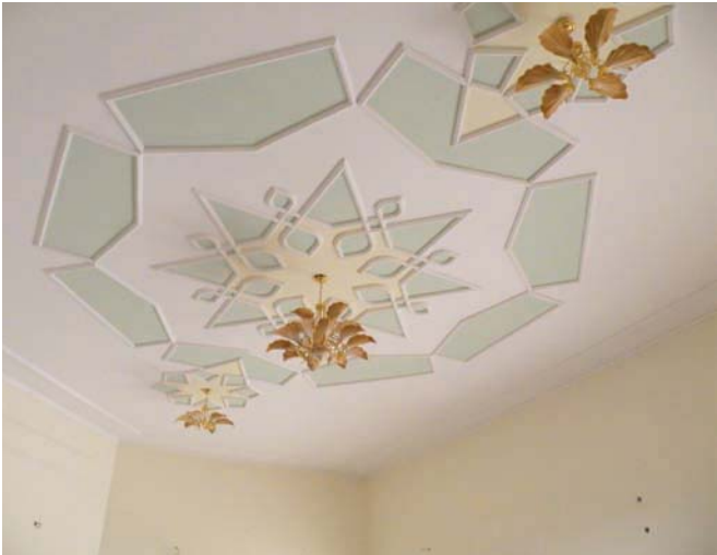
Newly installed chandeliers and painted ceiling.
