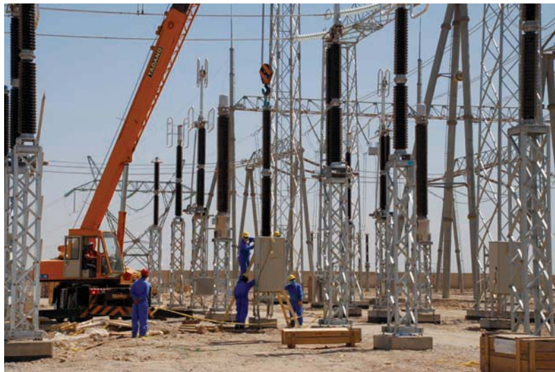
Qudas power plant. (USACE photo)
