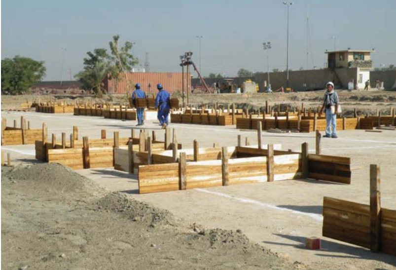
Contractors at work at the Anbar Rule of Law Complex.
