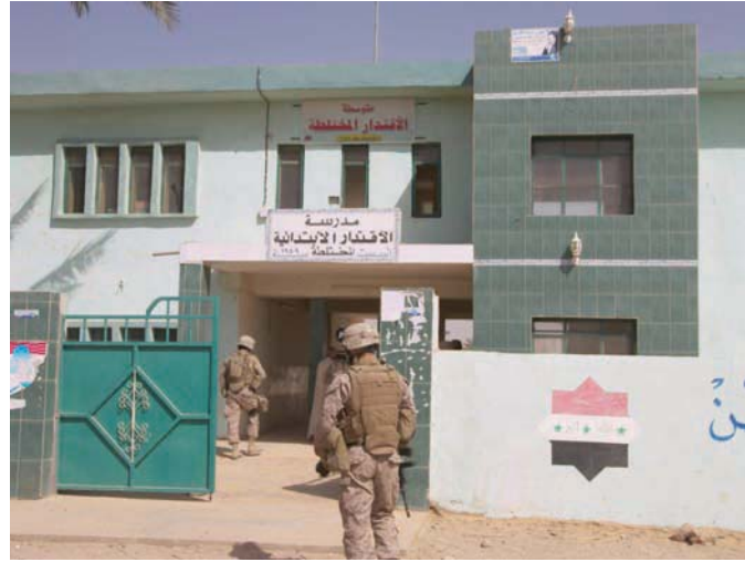
School exterior at time of SIGIR site visit.
