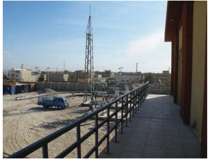
View from the substation building.
