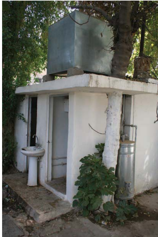
Photo of new latrine at Ninewa Provincial Police Headquarters.
