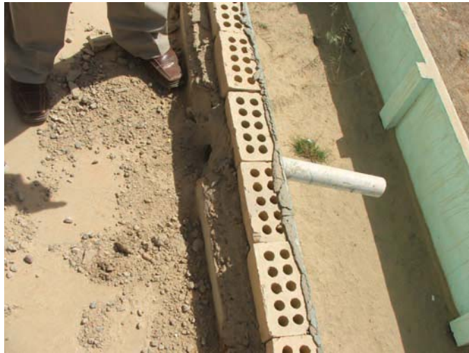
Drainage holes along roof edge.
