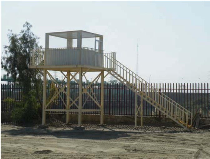
Guardhouse and fence.
