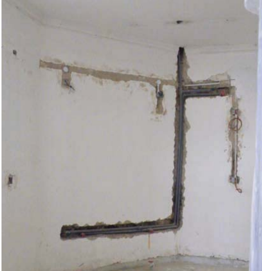
Partially completed interior finishing.
