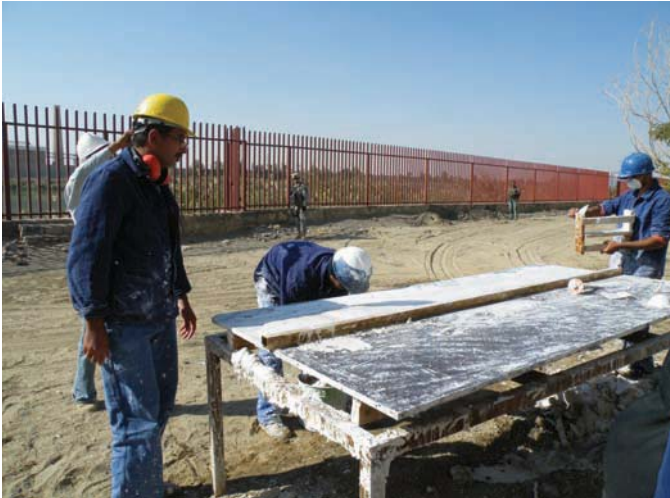
Contractors pouring molding for future installation.
