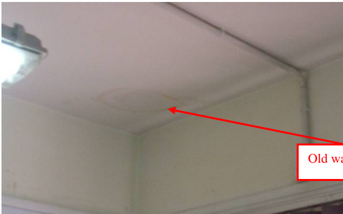
Site Photos 36 and 37. Old and dried out water spots on the ground floor Operations Room ceiling
