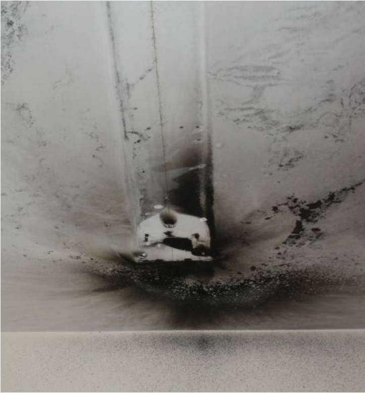
Site Photos 44 and 45. Electrical fire damage around the fluorescent light fixtures
