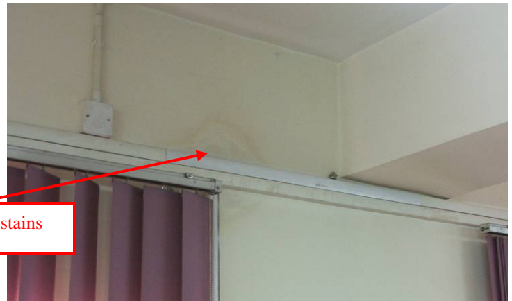
Site Photos 36 and 37. Old and dried out water spots on the ground floor Operations Room ceiling
