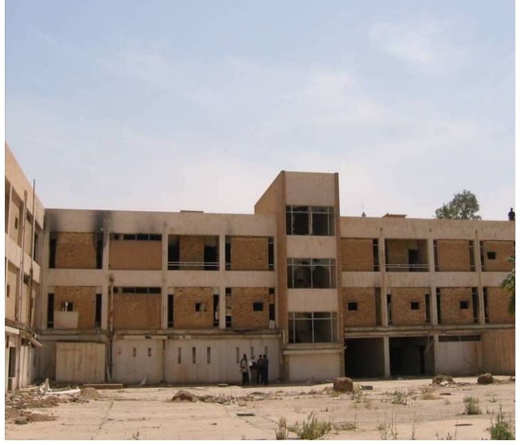
Site Photo 2. Exterior view prior to renovation (Photo courtesy of the USACE)
