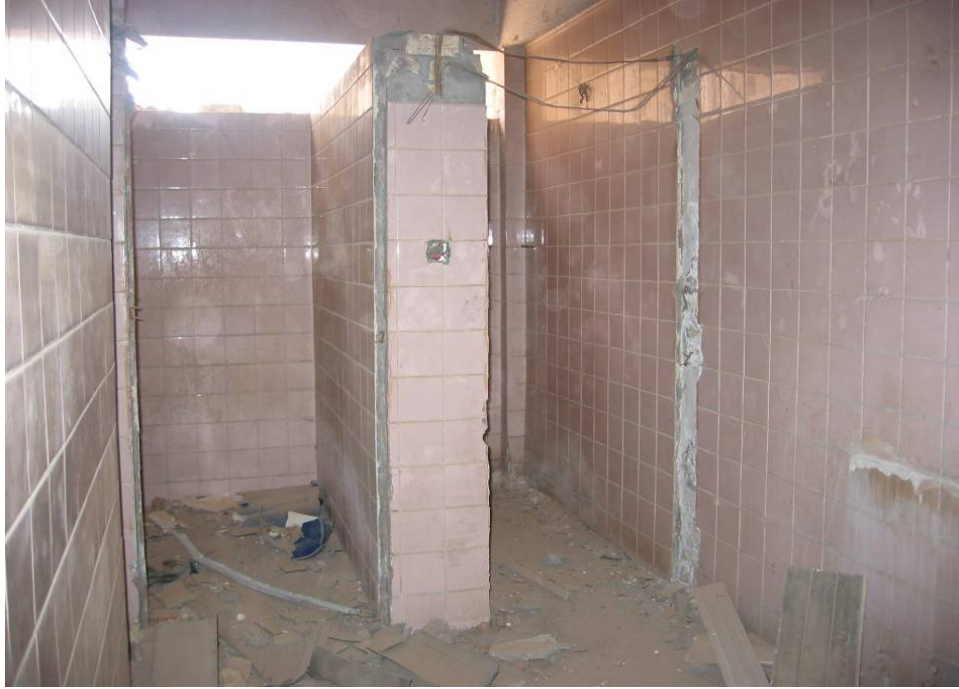
Site Photo 5. Condition of bathroom prior to renovation (Photo courtesy of the USACE)
