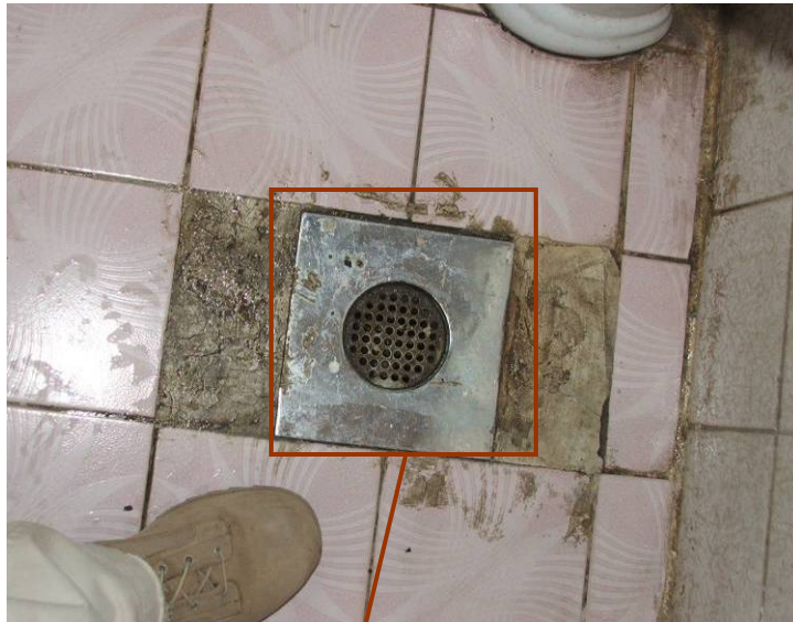
Site Photo 16. First floor bathroom floor drain
