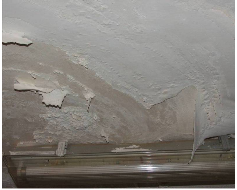
Site Photo 8. Additional view of water damage to ceiling (Photo courtesy of the USACE)
