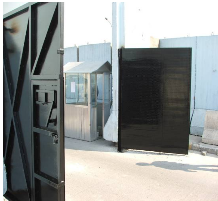
Site Photo 57. Manual gate installed by the ICD HQ
