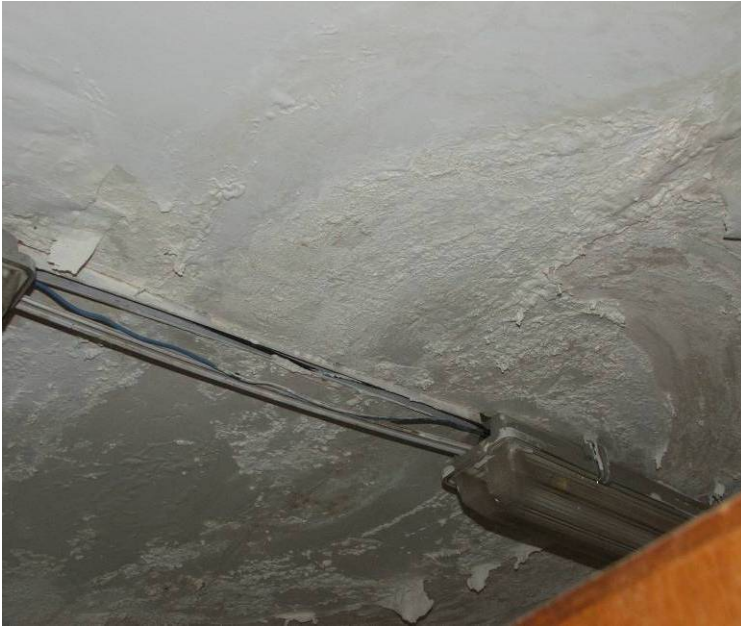
Site Photo 7. Water damage to ceiling of 1 st floor bathroom (Photo courtesy of the USACE)
