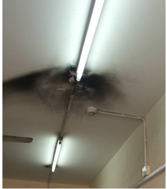
Site Photos 44 and 45. Electrical fire damage around the fluorescent light fixtures
