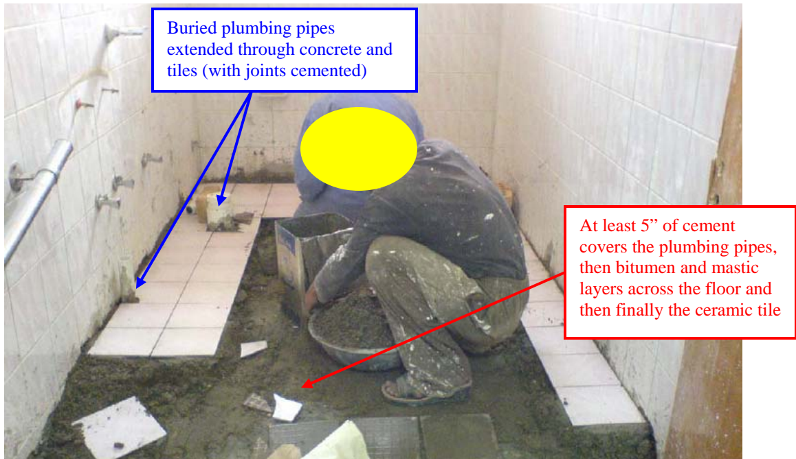
Site Photo 12. Bathroom after concrete has been poured and tile being applied (Photo courtesy of the USACE)
