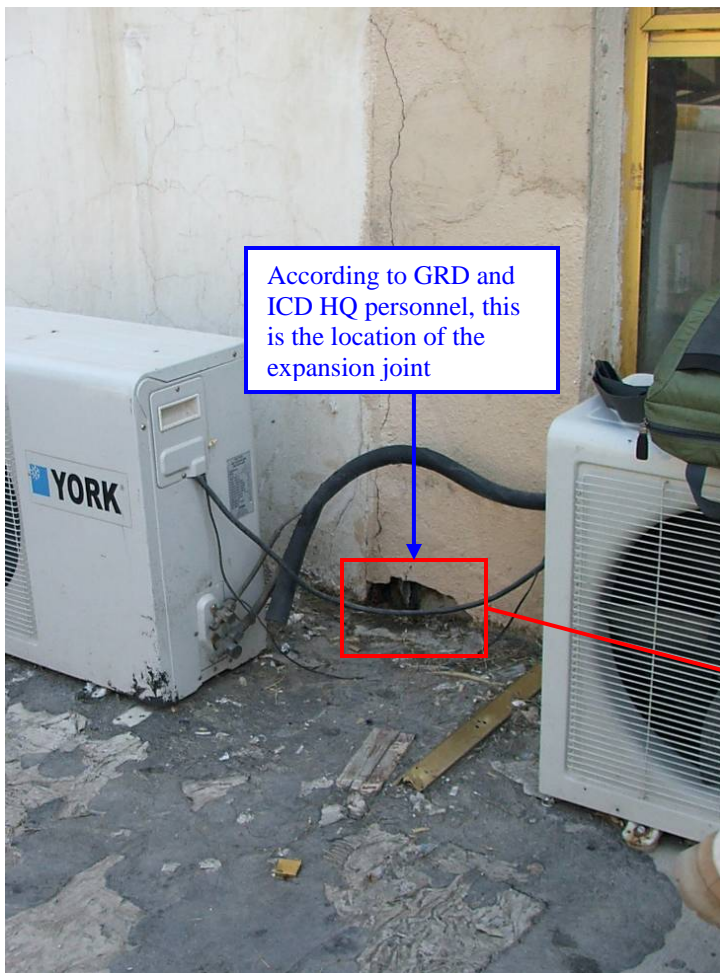
Site Photo 58. Location of the expansion joint
