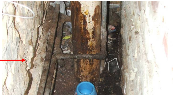
Site Photo 34. Close up view of bottom of Site Photo 32
