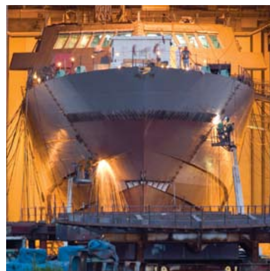
NMC is leading an effort to bring friction stir welding on site to the shipyard, allowing the Littoral Combat Ship to benefit from this process on a large scale for the first time. Lockheed Martin Corporation photo
