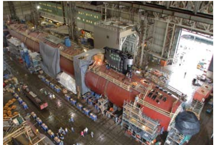
NMC has a number of new projects aimed at reducing labor hours and subsequent costs in the construction of the Virginia Class Submarine. General Dynamics Electric Boat photo
