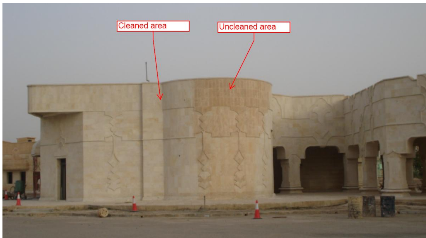
Site Photo 1. Example of renovation work – cleaning of the exterior building (Courtesy of USACE)
