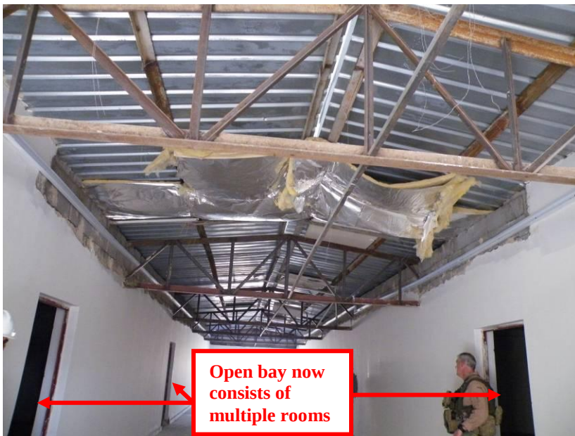
Site Photo 9. Interior view of training facility
