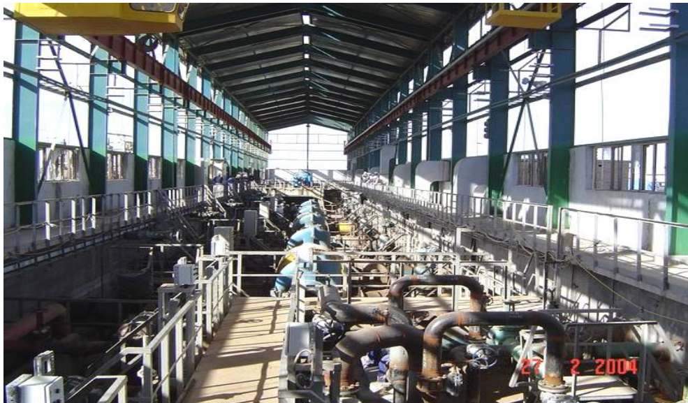
Figure 6—Ramallah Water Injection System After Repair
