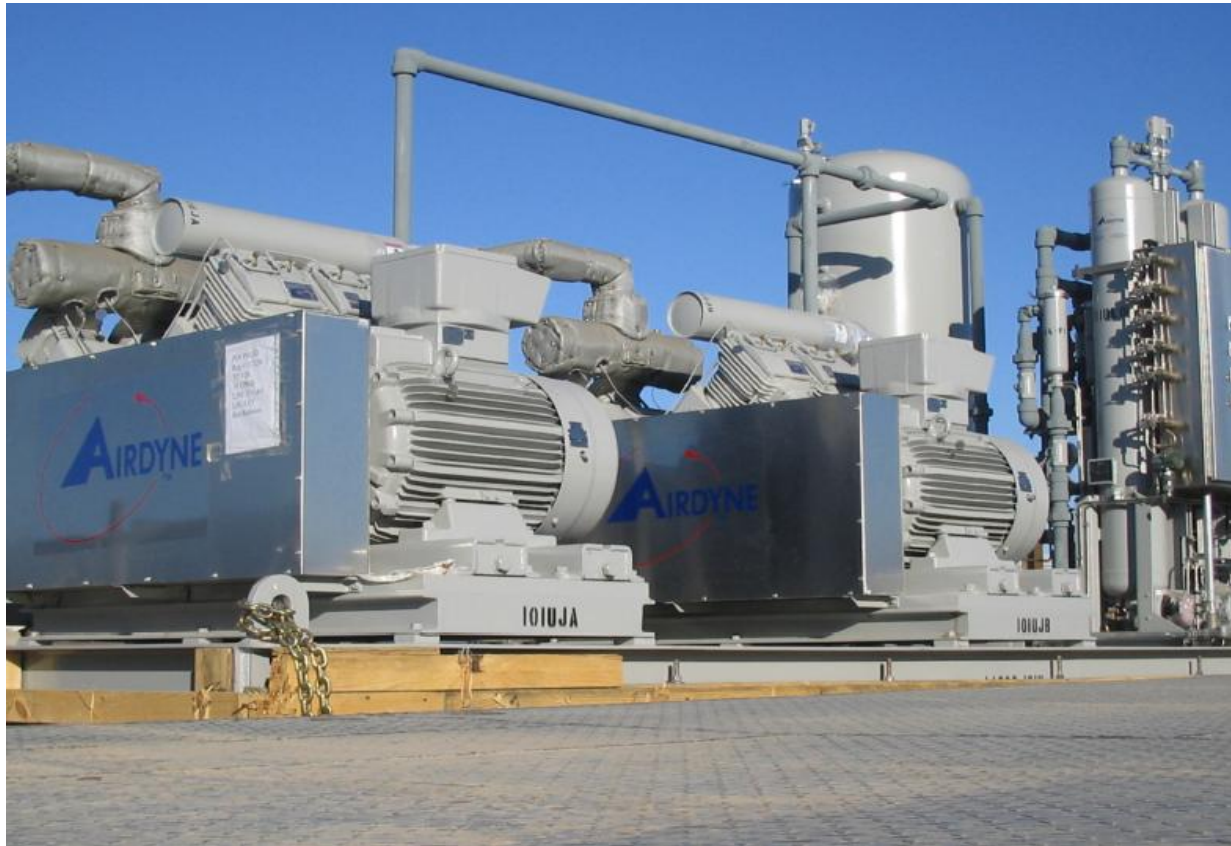
Figure 11—Task Order 20 - Compressor for Installation
