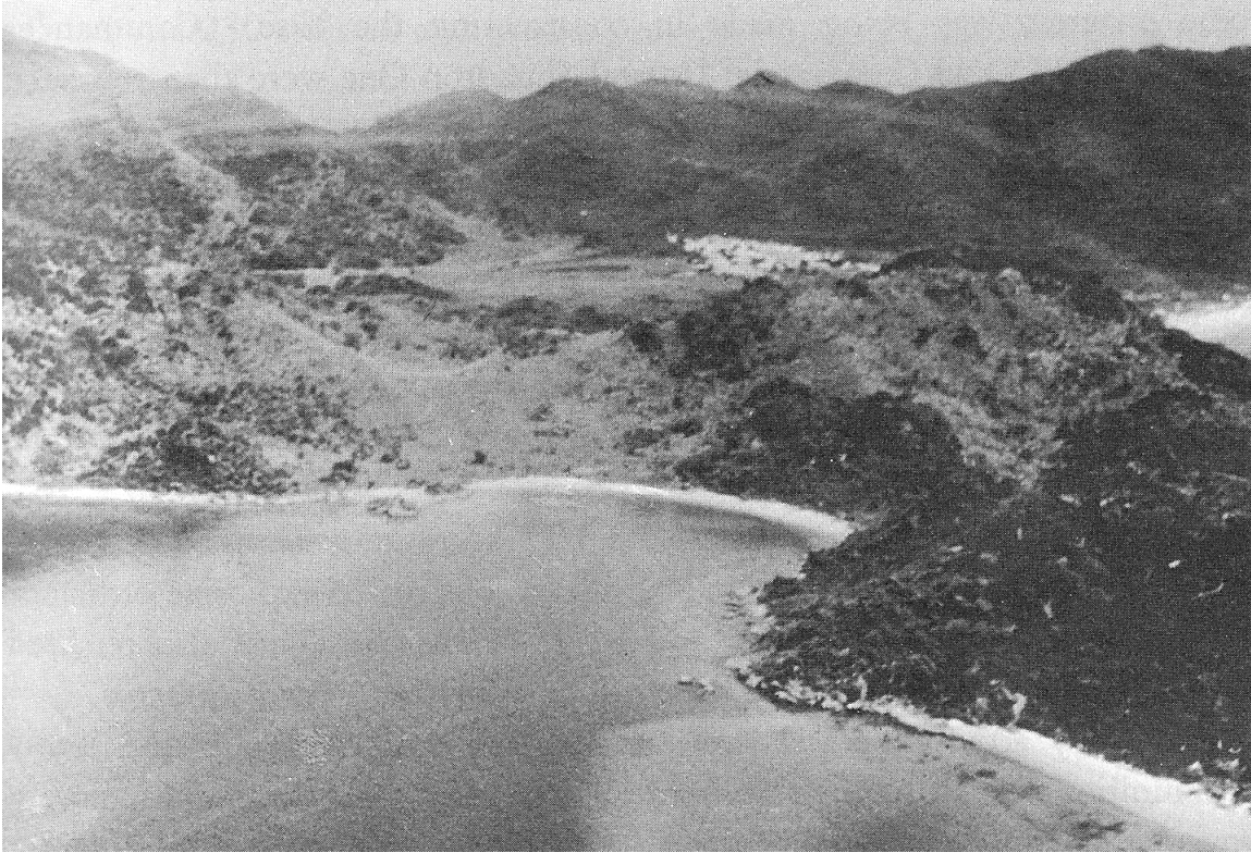
Figure 4. Cam Ranh Bay, 1965, before development as a logistical complex. (From [4] courtesy of the Naval Historical Center, Department of the Navy.)
