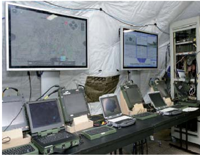
Figure 104. General Dynamics EDGE Facility (From General Dynamics, 2008)
