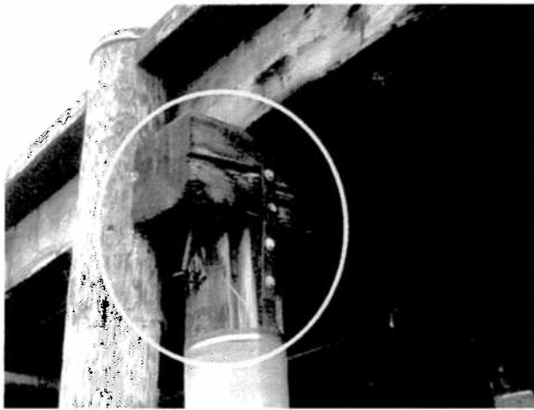
Figure 24 – Splintered pile at pile cap interface
