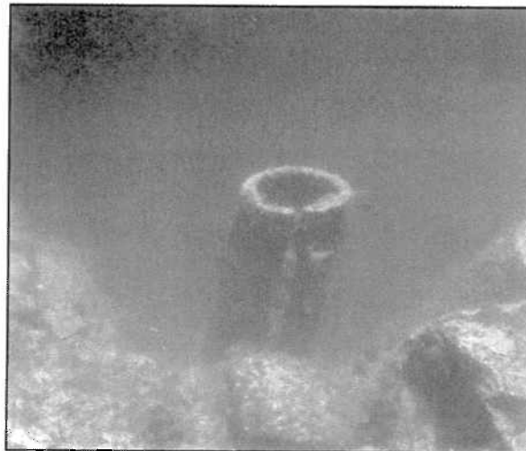
Figure 16 – Sample pile demonstrating potential for interior pile degradation
