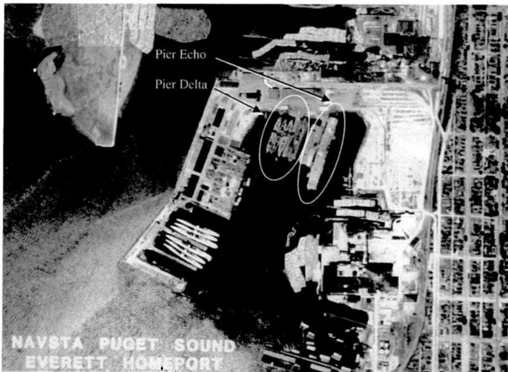
Figure 4 – Aerial view of NS Everett, circa 1946
