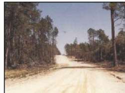
Typical clay surface Range roads. A well-maintained, heavily traveled road (above) in contrast to an example of a marginal road.
