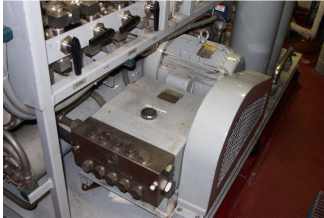
Figure 3-14: RO HP Pump and Motor with 3.6:1 Ratio V-belt Drive
