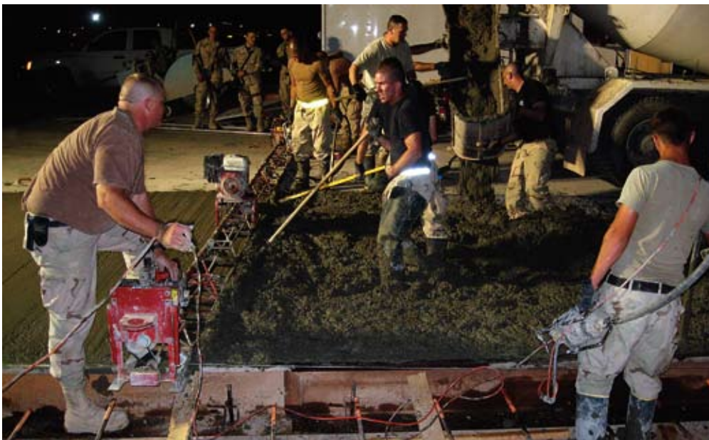
At Balad AB, pouring concrete at night lessens thermal stress on fresh concrete used for runway joint repair. (U.S. Air Force photo)
