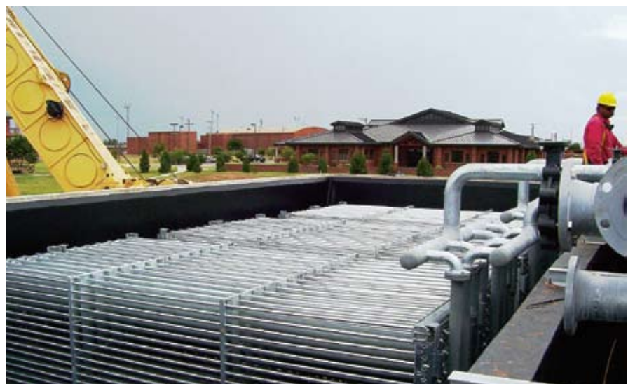
Built using an ESPC, Dyess AFB's ice plant cools 13 buildings on the Texas base by distributing water cooled by ice produced at night, when the temperatures are at their lowest. (U.S. Air Force photo)
