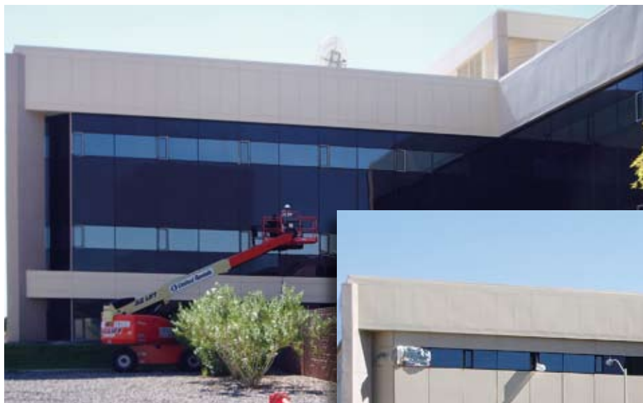
Glass spandrels (above) on Nellis AFB's Consolidated Support Facility "helped" raise the cooling load. Painting them over with a special ceramic coating (right) reduced the load and cooling costs. (U.S. Air Force photos)
