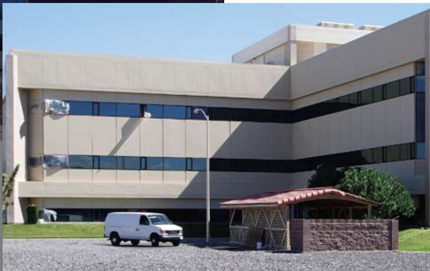
Glass spandrels (above) on Nellis AFB's Consolidated Support Facility "helped" raise the cooling load. Painting them over with a special ceramic coating (right) reduced the load and cooling costs. (U.S. Air Force photos)
