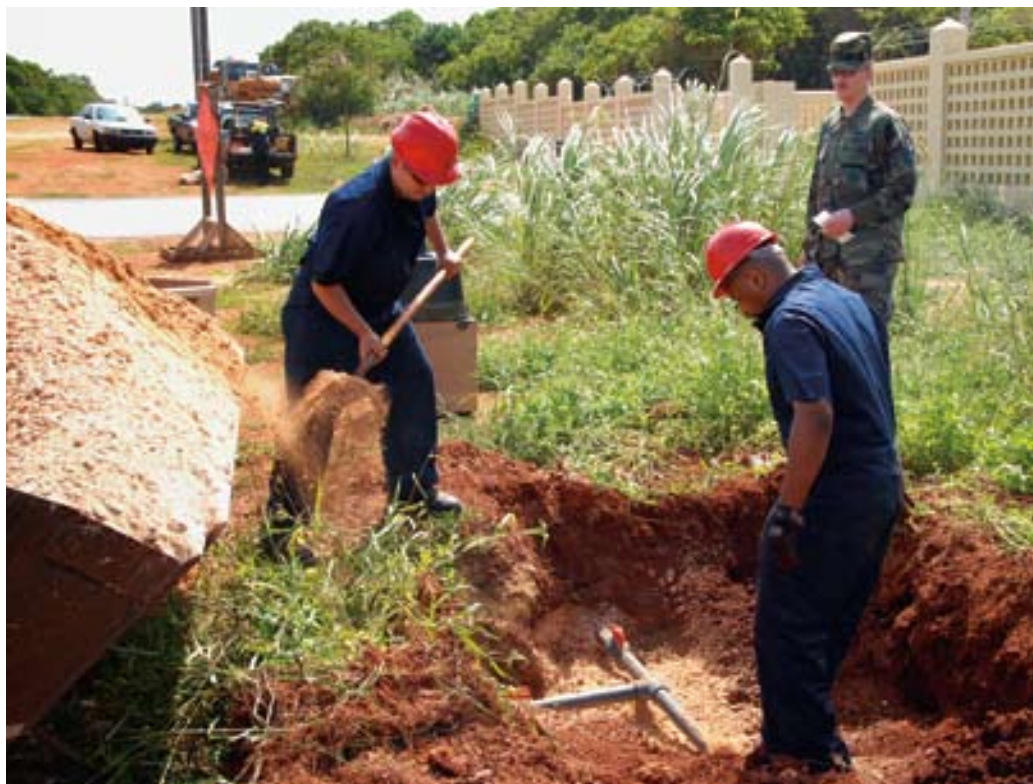
TSgt Jerry Hedstrom looks on as Tgt Todd McGee and TSgt Javier Vigil finish a new pipe and valve installation at the gate of Northwest Field, Guam. (photo by the author)
