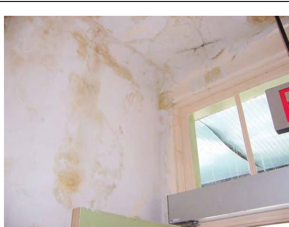
Building 4 – Partial or complete removal of plaster may be necessary; however, it is not recommended to replace a damaged plaster wall or ceiling with drywall. Fix the root cause of the problem before proceeding.
