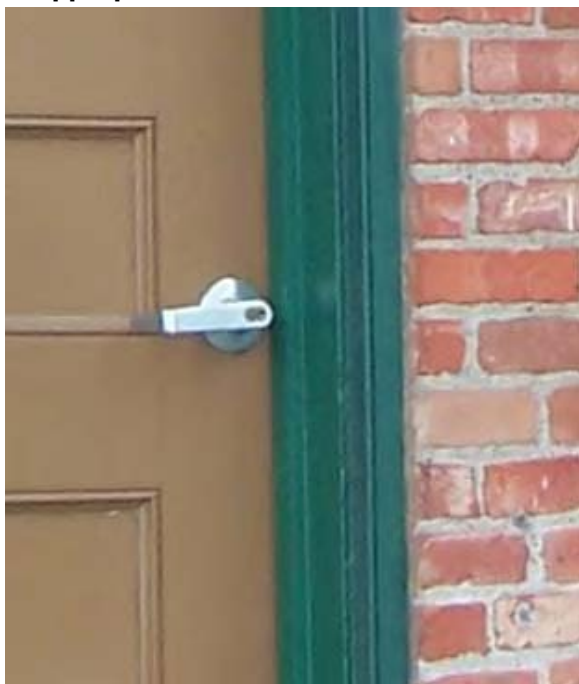
Building 128 – New lever door handle installed with compliance to the Americans with Disabilities Act (ADA).
