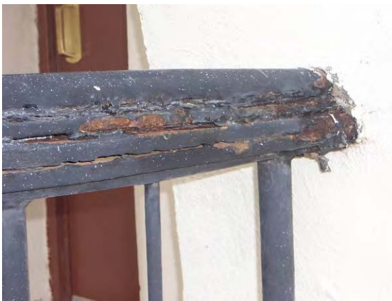
Building 315 – Close-up of the same metal railing above shows level of damage. Check for protective coating failure and identify cause of damage.
