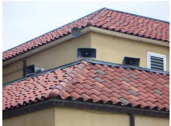
Building 311 – Overlapping clay roofing tiles.
