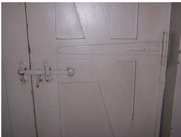
Building 54 – Original latch. Make sure that latch is not painted shut and is still operable.
