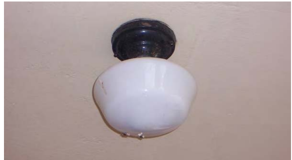
Building 515 – Original globe light fixture. Replacements should be in-kind to this style for interior light fixtures.
