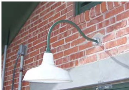
Building 613 – Good example of replacement exterior light fixture.
