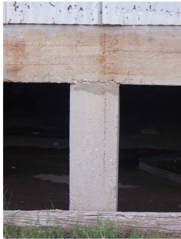
Building 1113 – Identify root cause of damage. Hairline, nonstructural cracks that show no signs of worsening normally need not be repaired. Cracks larger than hairline cracks, but less than approximately 1/16-inch, can be repaired with a mix of cement and water.
