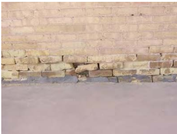
Building 13 – A periodic inspection of brick masonry should uncover damaged or deteriorated bricks. Deterioration and failure of brick near concrete foundation due to water damage.
