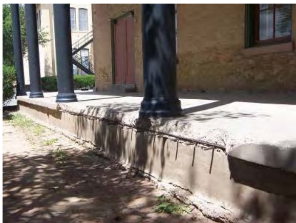
Building 13 – Repair the source of damage before repairing the concrete.
