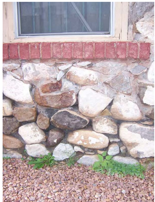
Building 2014 – Identify areas of missing mortar and loose stones.
