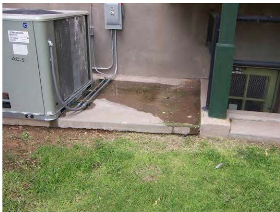
Building 1 – A periodic inspection will reveal areas of concern such as standing water on concrete.
