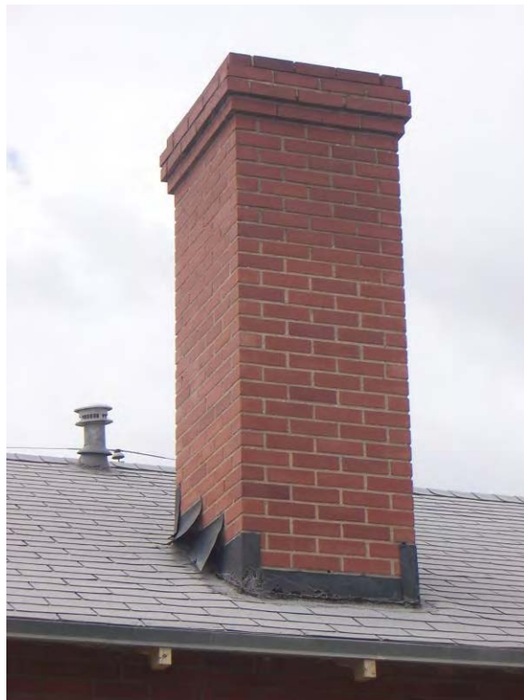
Building 612 – Example of improper use of step flashing. Be careful not to damage adjacent surfaces and materials such as chimneys and dormers when repairing the roof and flashing.
