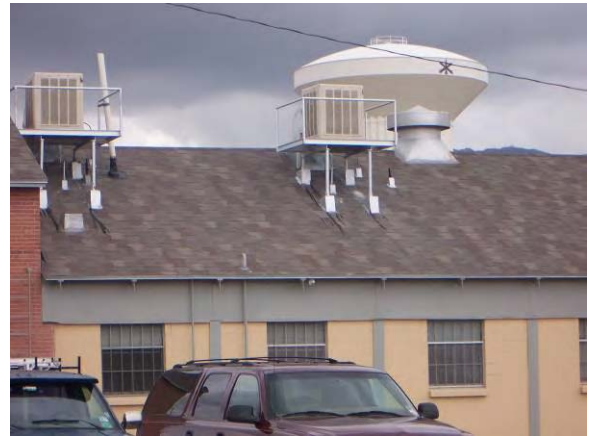
Building 641 – Multi-color interlock asphalt shingles.
