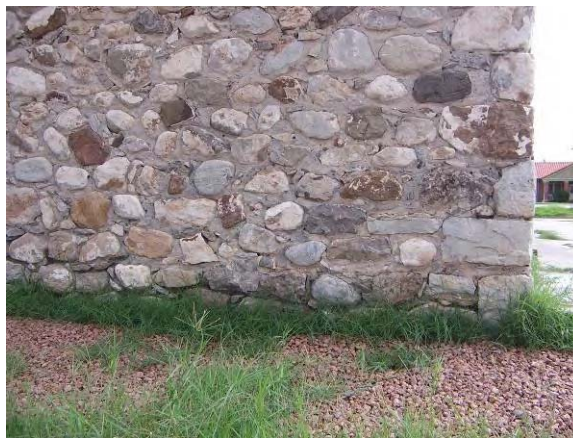
Building 2014 – This is a good example of a natural stone and mortar wall; however, the base of the wall needs to be inspected. Determine the repairs needed for the damaged stones and mortar at the base of the wall caused by water.
