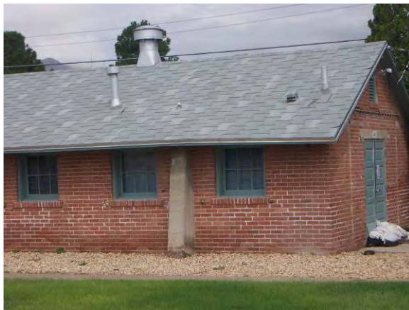
Building 440 – Gray interlock asphalt shingles.
