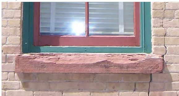
Building 13 – A periodic inspection of sandstone will reveal areas of damage. Identify areas of soft sandstone that are weathered and may need to be addressed.
