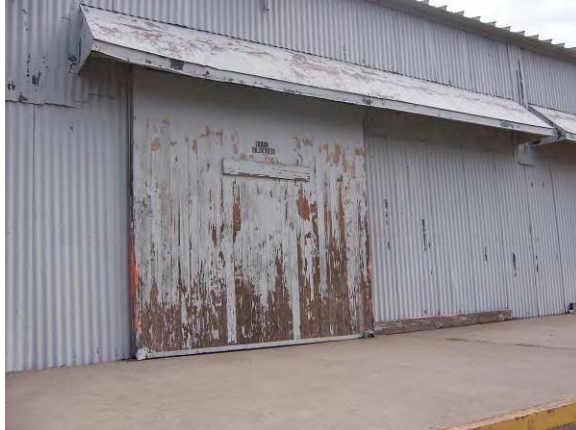
Building 1113 – Inspect the original wood sliding door to see if it is still operable, the condition of the paint, and the soundness of the overall door and track system.
