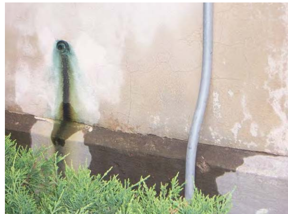
Building 243 – Inspect areas of concern such as visible water on stucco surfaces.
