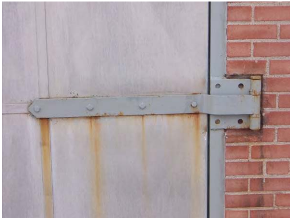
Building 624 – Mixing different metal types will lead to galvanic corrosion to metal hardware, in this case, the door hinge.
