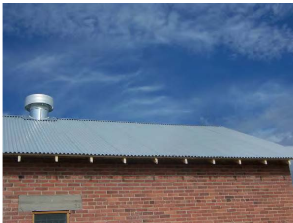
Building 889 – Crimped metal roof.
