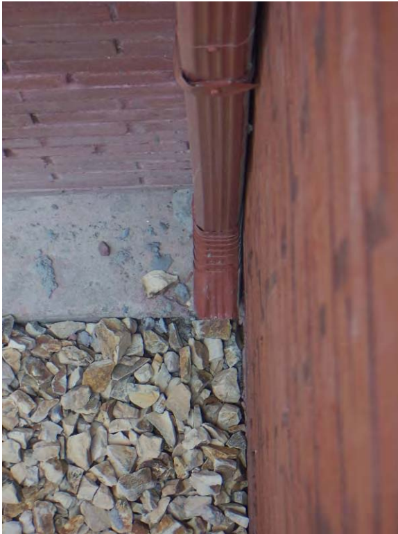
Building 4 – Stones are a good example of erosion control; however, the water from a downspout should flow into a downspout extender that transports water at least 3 feet from the foundation.
