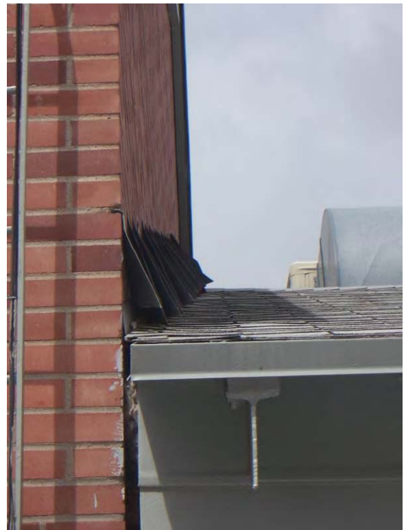
Building 620 – Stepped flashing that has become detached. Also there is no gutter installed to help transport water away from the building, especially the large gap in between the two walls and roof.
