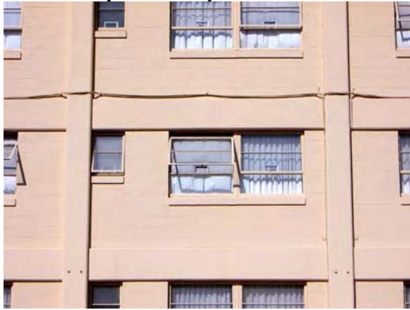
Building 5015 – Make sure that original metal windows are operable and that they have not been painted shut.
