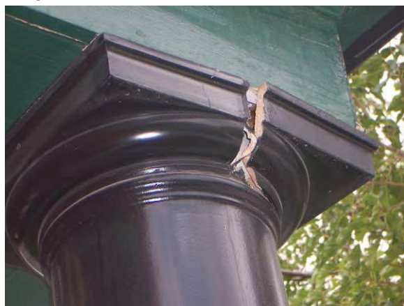
Building 4 – A periodic inspection of buildings would reveal damaged features such as this wood capital.
