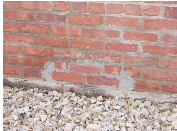
Building 442 – Inappropriate mortar patching. Determine a mortar mix that is chemically and visually compatible to the building and existing materials.
