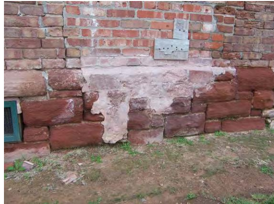
Building 128 – High-pressure water blasting or sandblasting is NOT recommended to clean efflorescence off of brick.
