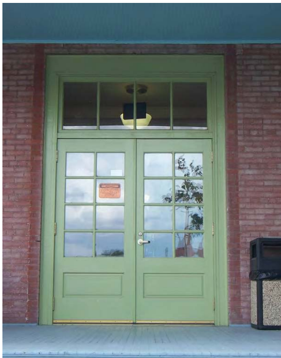
Building 4 – Appropriate replacement wood and divided light doors and transom but not appropriate door hardware.
