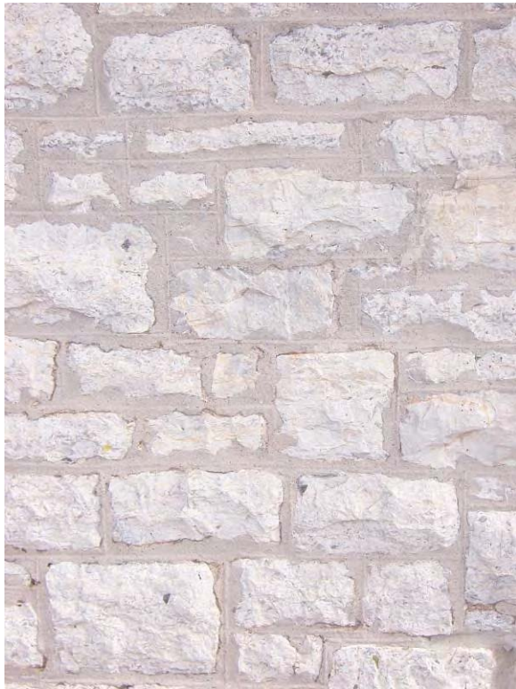
Building 2009 – Removing non-deteriorated mortar from sound joints, and then repointing the entire building to achieve a uniform appearance is not recommended.
