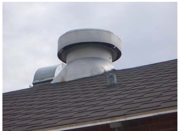
Building 624 – Original metal roof ventilator. Regular inspection and maintenance should be done on all roof/ventilation equipment.
