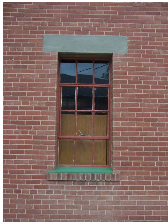
Building 54 – Metal divided-light awning window.
