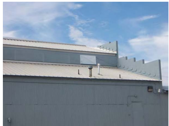
Building 1008 – Metal channel roof.
