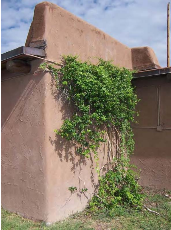
Building 5041 – Vegetation should not be allowed to grow on the stucco wall. Lack of proper maintenance increases the likelihood of problems that can lead to the breakdown of the stucco skin.
