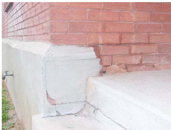
Building 111 – Patch and repair damaged concrete with a material similar or compatible to the original material in color and texture.
