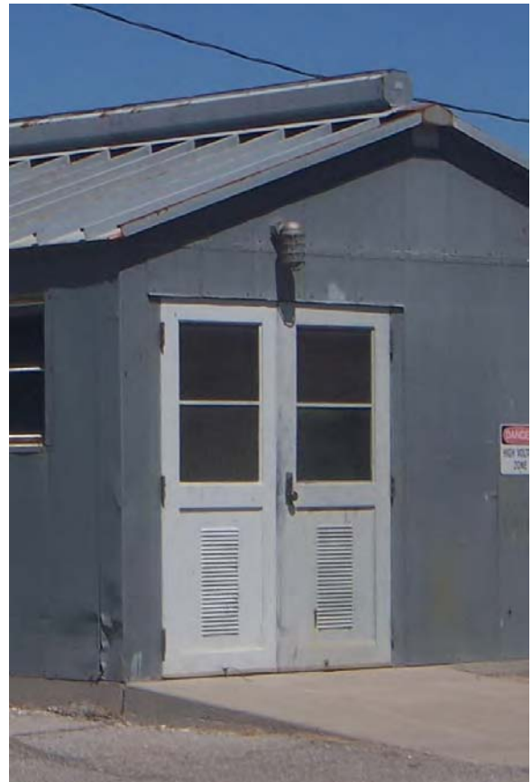
Building 742 – The evaluation of original metal doors should include a test for the presence of corrosion, overall condition of the paint, and the presence and condition of hardware. Note where original hardware is intact.
