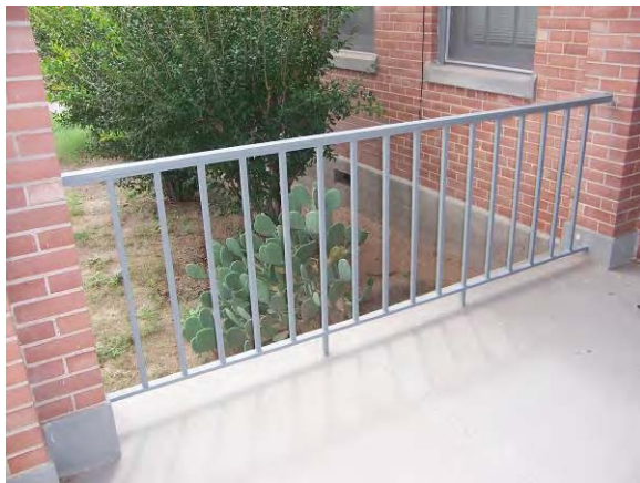
Building 629 – Clean architectural metals when necessary, to remove corrosion prior to repainting or applying other appropriate protective coatings.
