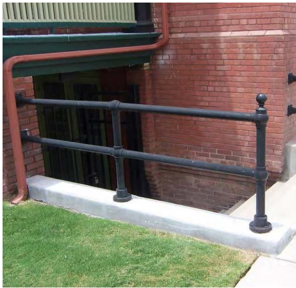
Building 4 – This metal handrail is a good example of replacement in-kind to the original metal feature.
