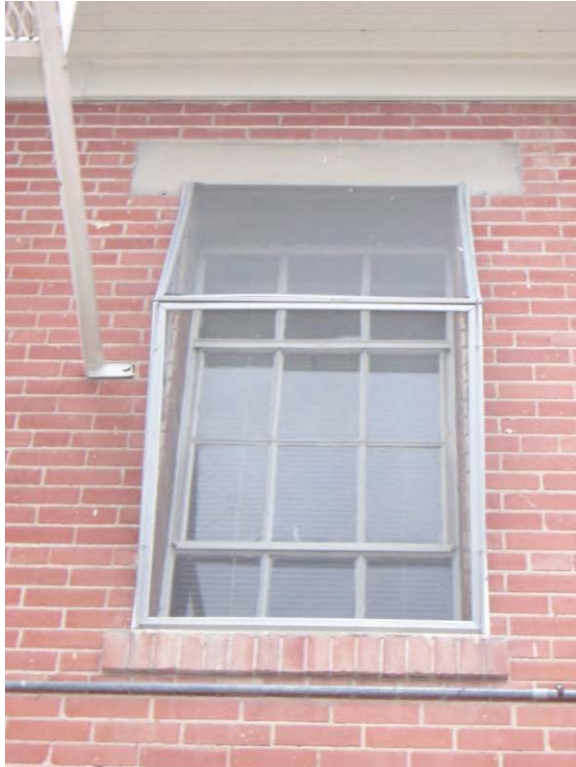
Building 54 – This is an inappropriate metal screen placed over a metal awning window. The screen needs to be removed.
