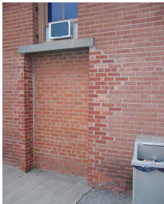
Building 55 – This is an appropriate infill of a door opening since it is recessed and exhibits similar shadows of the original opening. However, the brick type and mortar mixture used around the opening are not appropriate to the building type.
