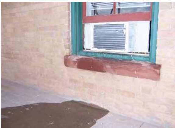
Building 13 – Areas of spalled sandstone caused by water damage should be identified. Water dripping from the window air conditioning unit is damaging the sandstone windowsill. Determine whether the sandstone piece can be repaired through patching or if the piece needs to be replaced.
