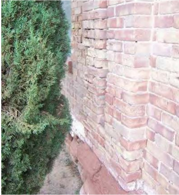
Building 128 – Brick deterioration due to the proximity of vegetation to the brick exterior wall.
