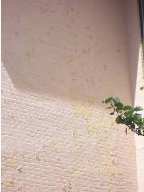
Building 21 – Remove damaged or deteriorated paint only to the next sound layer using the gentlest method possible (e.g., hand-scraping) prior to repainting. Apply compatible paint coating systems following proper surface preparation, and paint with colors that are appropriate to the historic building and district.
