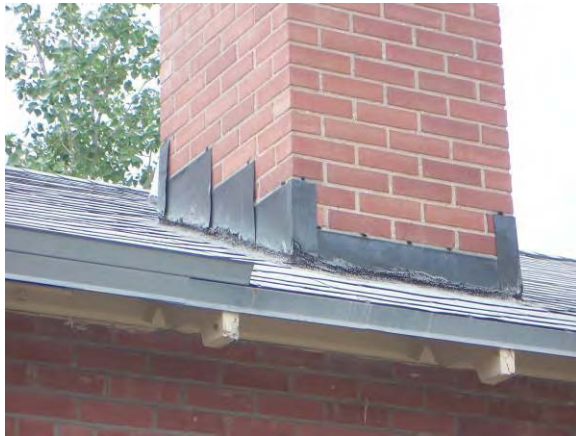
Building 612 – Correctly installed flashing detail around chimney base.
