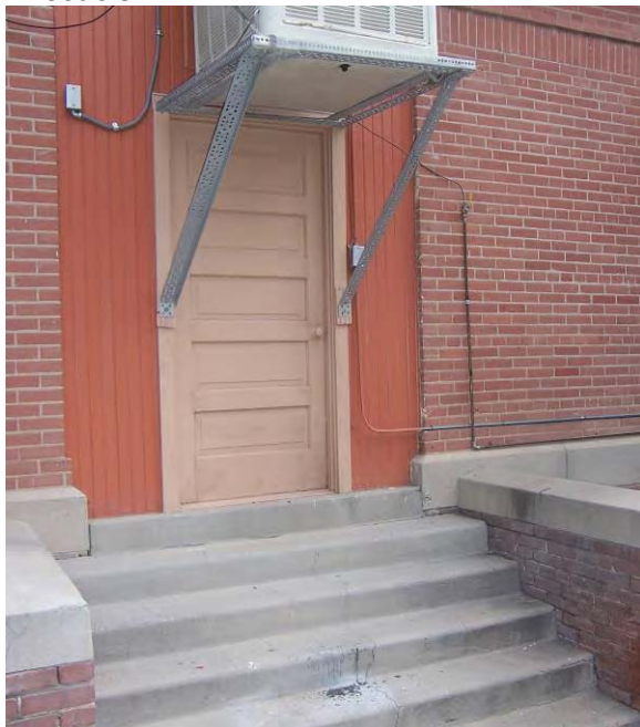
Building 55 – This is an inappropriate placement of an evaporative cooler.
