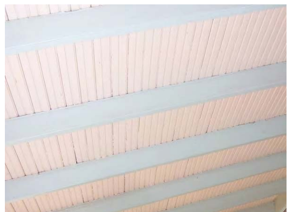
Building 13 – Beadboard and exposed rafters are character-defining features of some Fort Bliss buildings.
