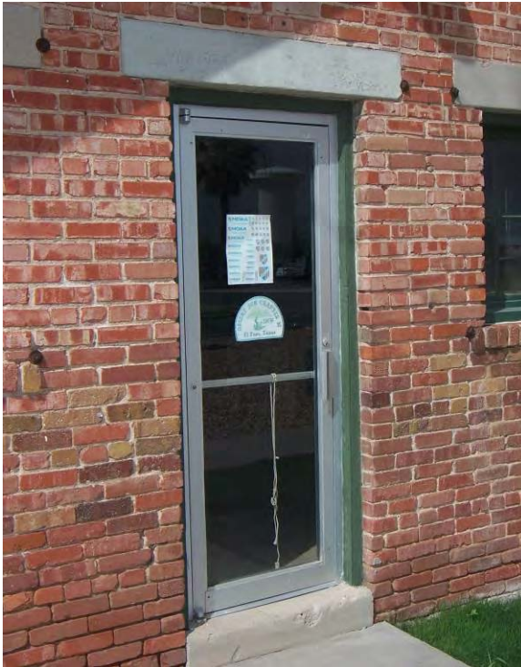
Building 442 – The bright aluminum and plate glass door replacement is inappropriate and does not match the existing wood door style on the building. However, the original wood door frame is still intact.
