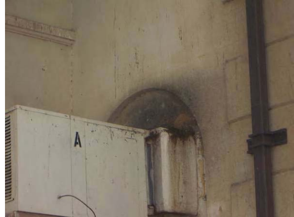
Building 243 – Inspect and determine if the stucco needs to be cleaned to maintain and preserve the material.
