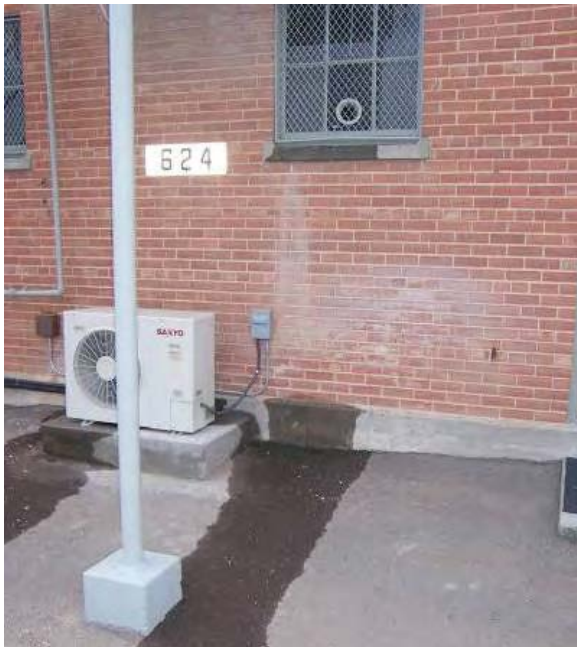
Building 624 – Identify the source of damage. Water is constantly running down the surface of the brick exterior wall from the evaporative cooler located above the window.
