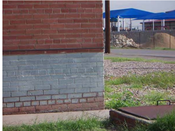
Building 122 – Do not paint historic surface materials that were originally not painted.
