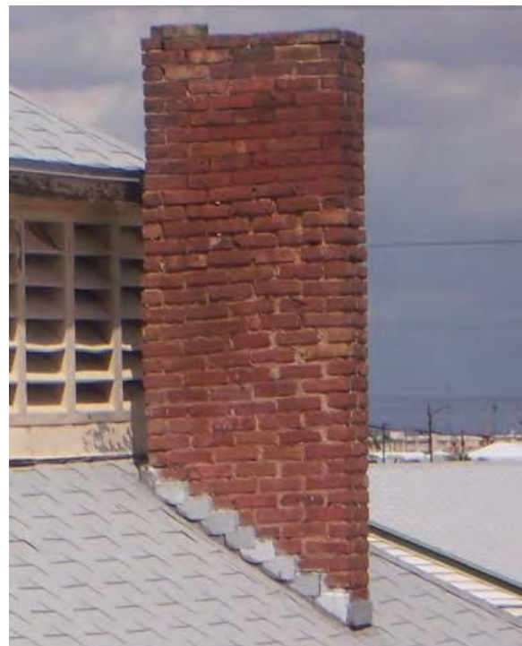
Building 19 – Untreated brick and mortar failure may lead to chimney failure.
