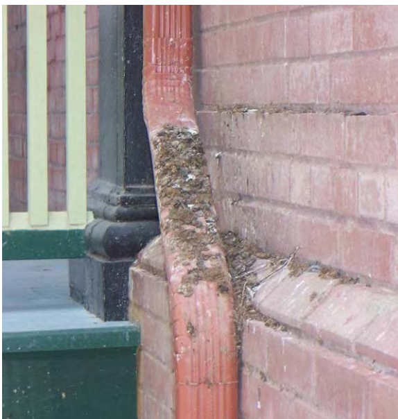
Building 4 – Although the gutter is not historic, proper removal of pigeon guano should be maintained since the gutter is part of a historic building. Do not use bleach on bird guano.
