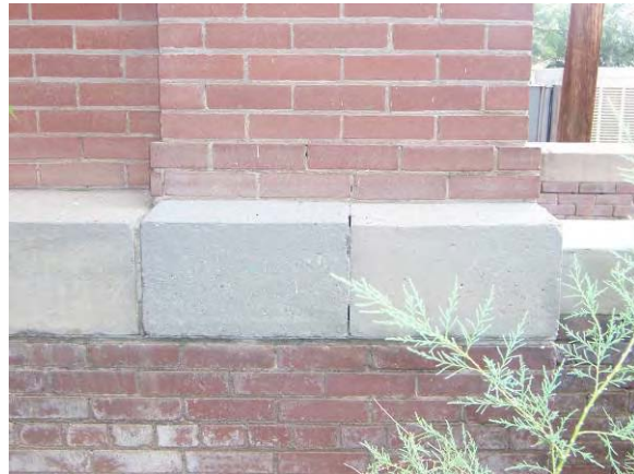
Building 55 – Exposed concrete water table detail.
