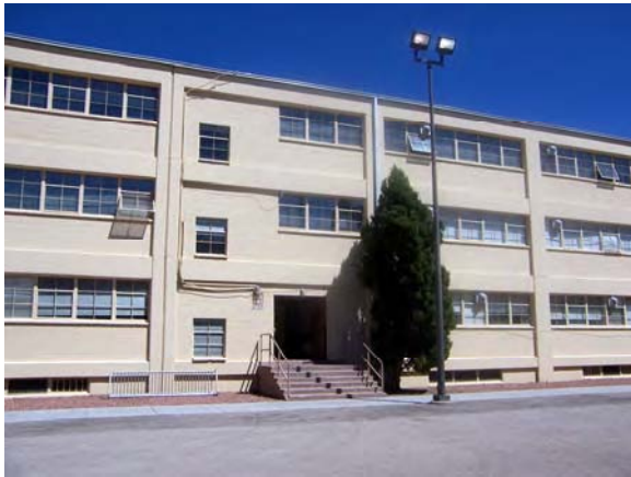
Building 1002 – Painted concrete block exterior walls with concrete framework.
