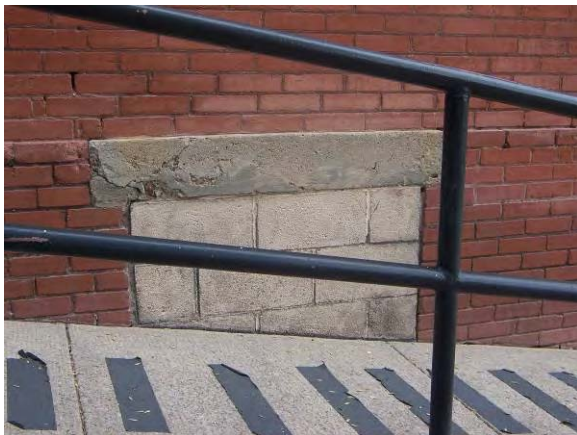
Building 1 – An ADA access ramp blocks the inappropriate concrete block infill of a window opening.
