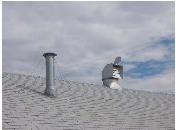
Building 444 – Gray three-tab asphalt shingles.
