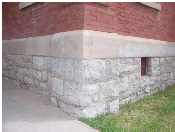
Building 51 – Natural stone was typically used in foundation walls.
