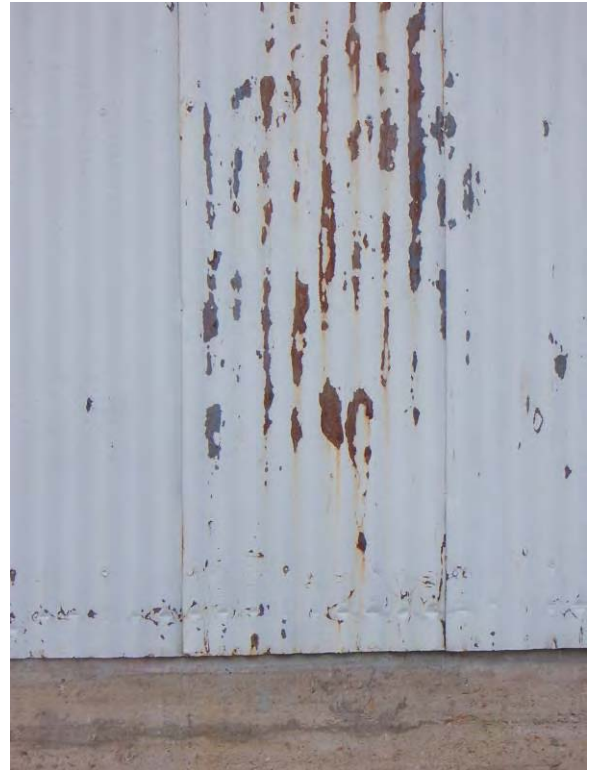
Building 1113 – Determine the cause for the chipping paint and rust and prescribe the proper procedure for repair of the metal element.
