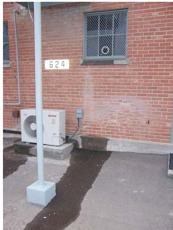
Building 624 – The water is constantly dripping onto the concrete foundation and windowsill from the air conditioning units.
