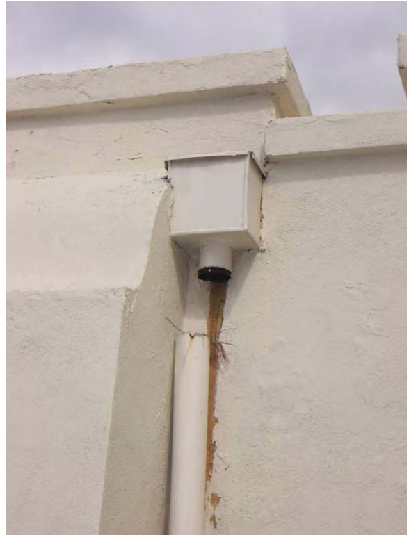
Building 315 – Downspouts, flashing, leaders, roof drains, and scuppers are all part of the drainage system, and should be included in the work list when maintenance or repairs are being inspected and evaluated.
