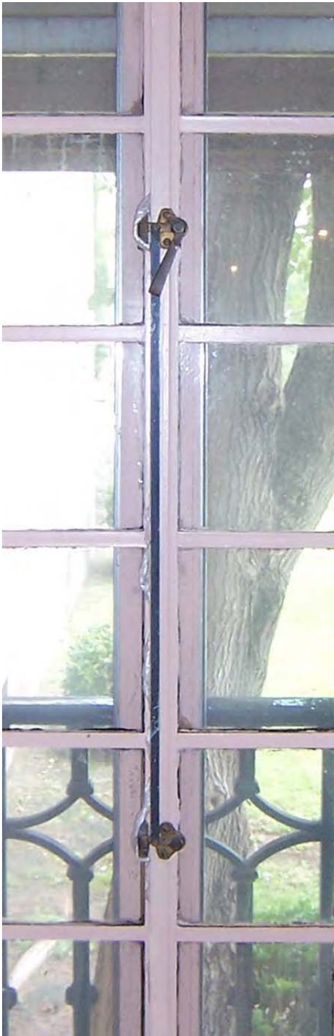
Building 243 – Brass and bronze hardware should not be painted. Clean original hardware with appropriate materials and regularly lubricate locks and hinges.
