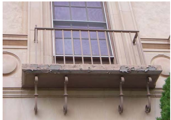
Building 504 – Inspection of this concrete canopy and metal railing show signs of deterioration. Need to protect and maintain architectural metals from corrosion by providing proper drainage so that water does not stand on flat surfaces such as the balcony.
