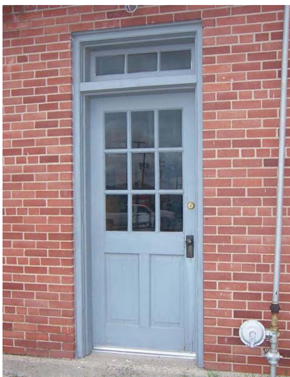
Building 613 – Original wood panel and divided light door with both original hardware and a new deadbolt.
