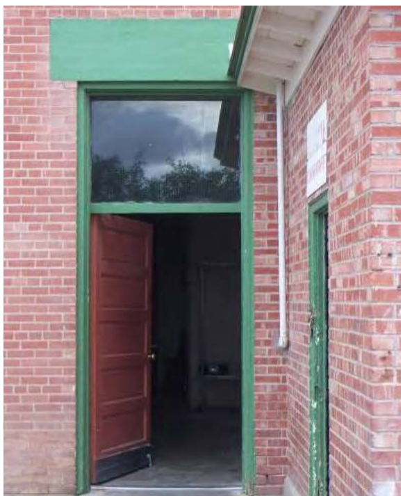
Building 54 – The replacement single-pane fixed transom above the door is not in-kind to the historic material of the building.
