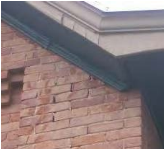
Building 128 – An inspection of brick walls will identify missing or deteriorated mortar.
