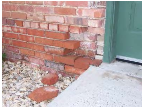
Building 442 – Bricks located near the foundation of a structure are susceptible to deterioration. Identify root cause of damage, including standing water.
