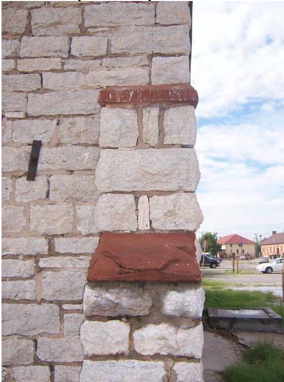
Building 2011 – Evaluate the condition of the mortar and sandstone. Both elements could lead to moisture problems for the natural stone.
