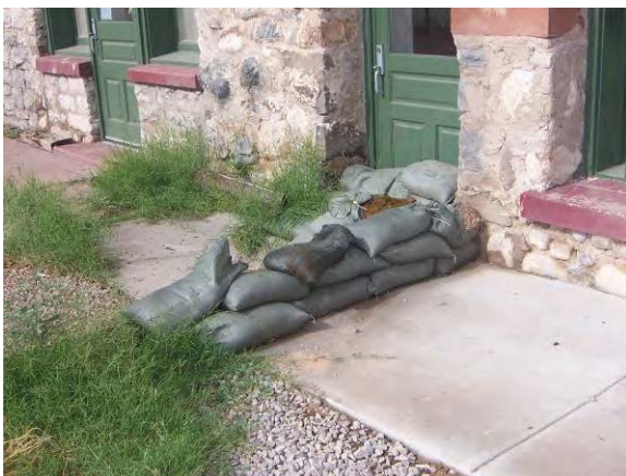
Building 2011 – Proper drainage is a key to maintaining stone and mortar foundation walls. An inspection found standing water near the foundation and door. Sandbags are not a permanent solution to the problem.
