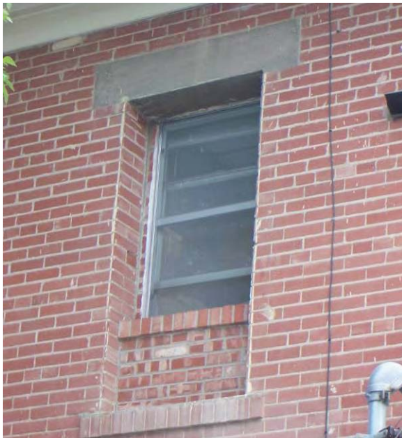
Building 54 – Poor example of window replacement. It is not recommended to modify a window opening as shown above. The replacement window should be in-kind to the original
