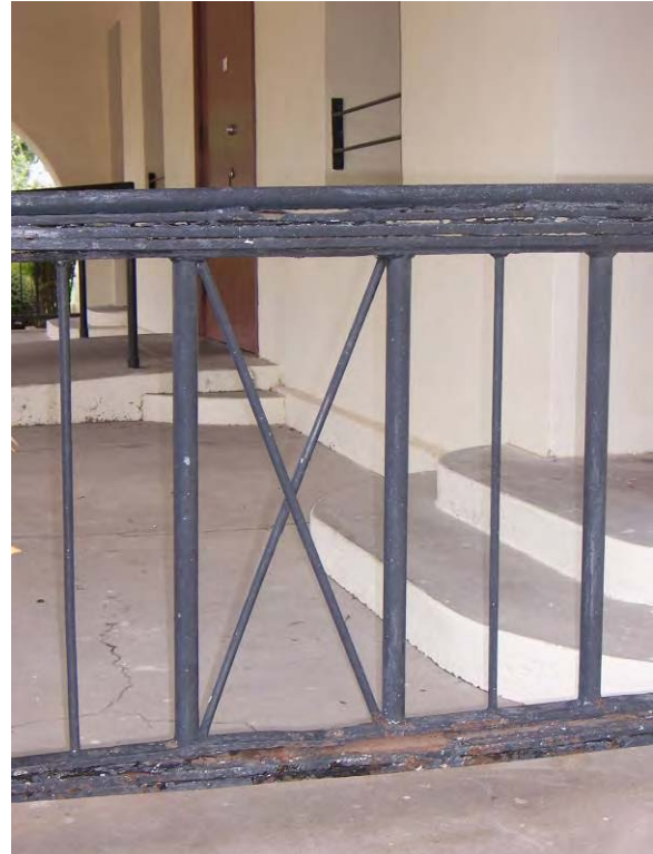
Building 315 – Surfaces of raw metal should be examined for signs of rusting. Provide an appropriate protective coating.
