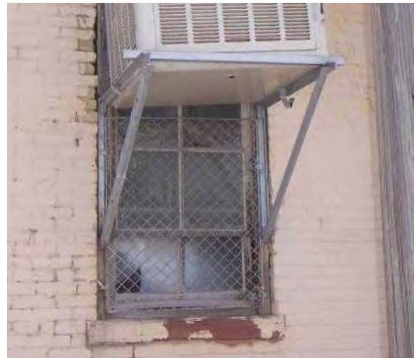
Building 21 – Evaluate the condition of the sandstone feature and repair source of damage before repairing sandstone. Do NOT apply paint to sandstone that was historically unpainted.
