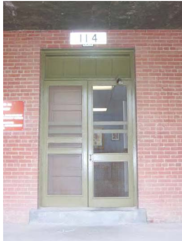
Building 114 – Determine original screen door style before replacing. Replacement wooden screen doors should match those original to the building.
