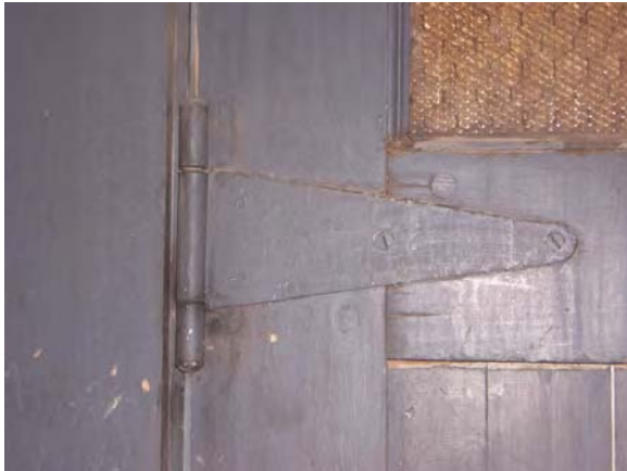
Building 7133 – Make sure all door hardware is properly secured to the frame and to the door.
