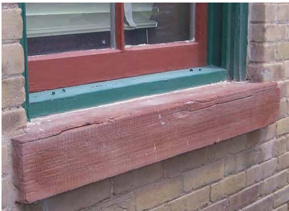
Building 13 – A periodic inspection of sandstone masonry should uncover cracking or spalling issues. The top of the sandstone windowsill is damaged from rain water standing on the flat surface.
