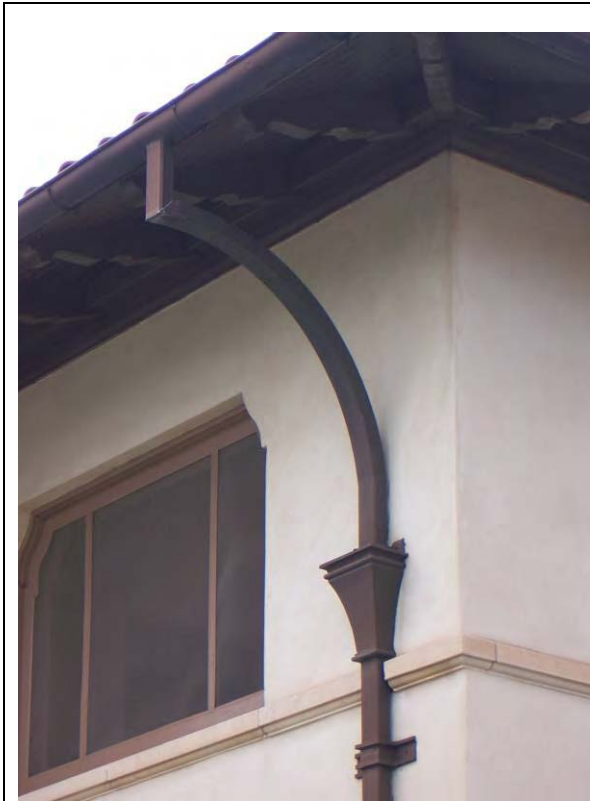
Building 243 – Decorative gutter and downspout.
