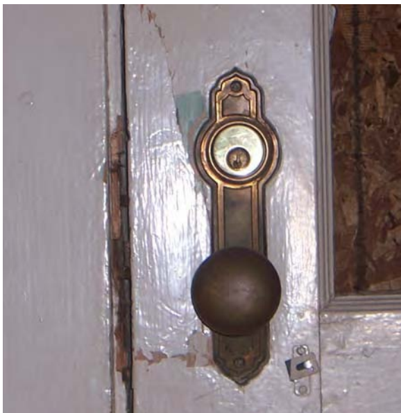
Building 7000 – Original decorative brass doorknob and lockset combination. Appropriate cleaning methods need to be used to preserve the hardware.
