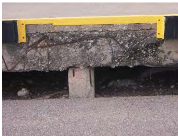
Building 1119 – Remove the concrete at spalled areas to expose the corroded steel bars. Once the deteriorated concrete has been removed, rust on the exposed rebars must be removed by wire brush. Note: If the rebars are so corroded that a structural engineer determines they should be replaced, new supplemental rebars will normally be required.
