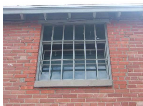
Building 624 – Evaluate the condition of the infill bricks and mortar. They should be in-kind to the existing bricks and mortar.
