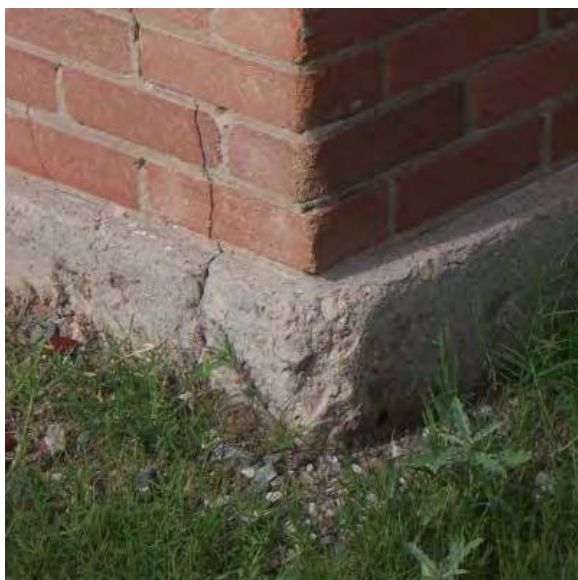
Building 889 – Provide proper water drainage away from concrete foundations so that water does not accelerate concrete deterioration.
