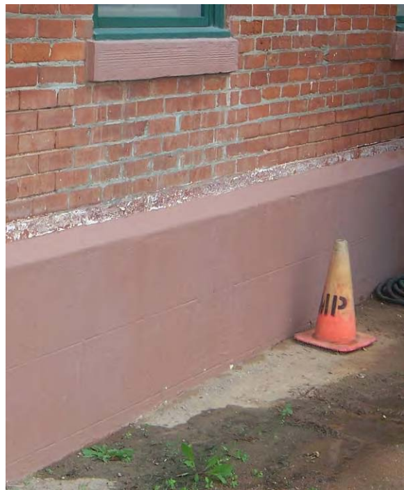
Building 128 – Painted and scored concrete foundation wall.
