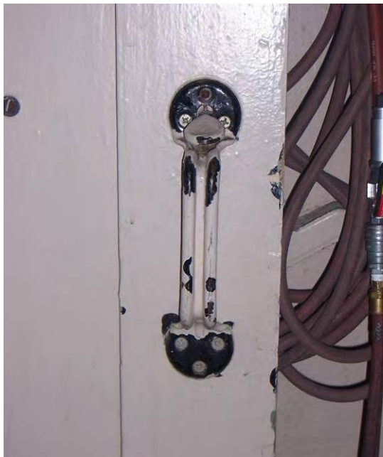
Building 54 – Peeling paint on historic hardware needs to be inspected and maintained.
