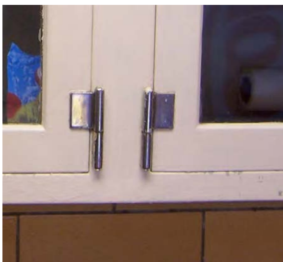
Building 7115 – A different set of metal hinges on wood cabinet doors.
