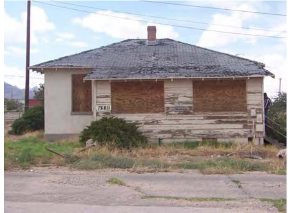
Building 7183 – Remove paint to the next sound layer by using the gentlest method possible (e.g., handscraping). DO NOT sandblast the wood to remove paint, which could damage the wood and drive moisture into the building.
