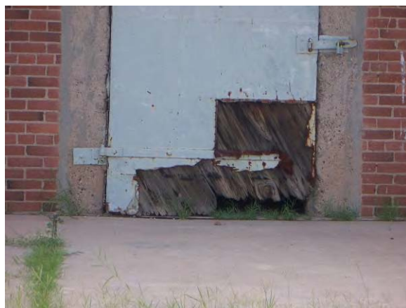
Building 888 – Need to inspect and evaluate the overall condition of the wood feature to determine whether more than protection and maintenance are required.
