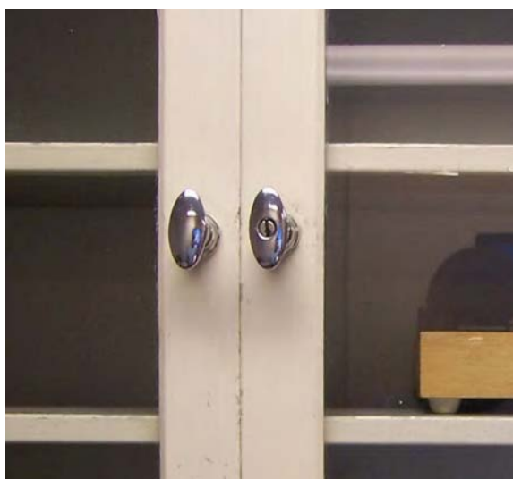
Building 7115 – Cabinet knobs with a lockset.
