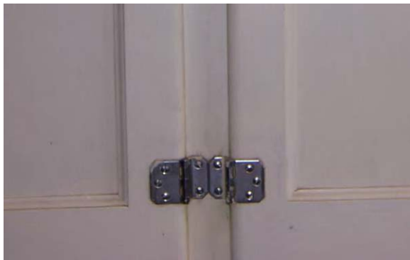
Building 504 – Metal cabinet door hinges
