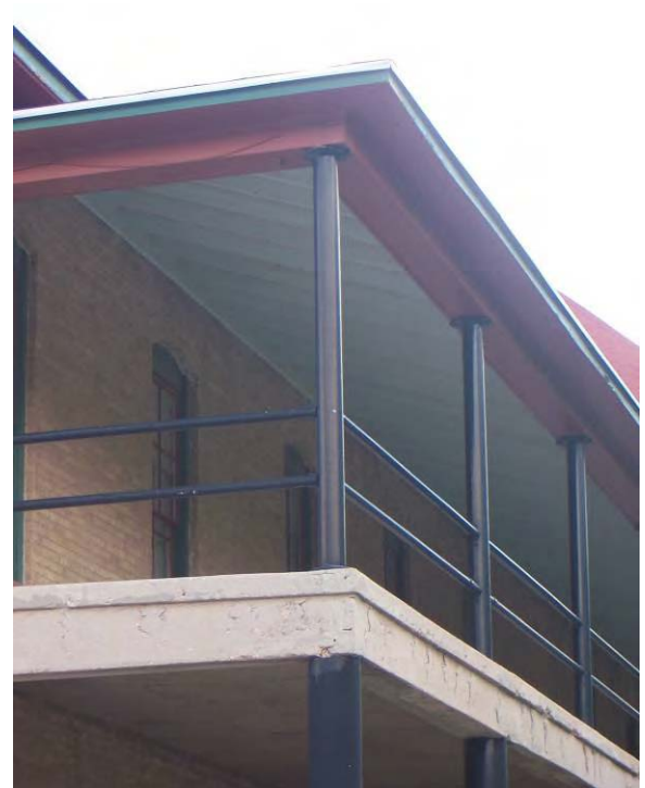
Building 13 – The metal columns and railings are in great condition. These elements in combination to the openness of the two-story balcony are integral features to the overall design of the building. They should be checked regularly for damage or maintenance requirements.
