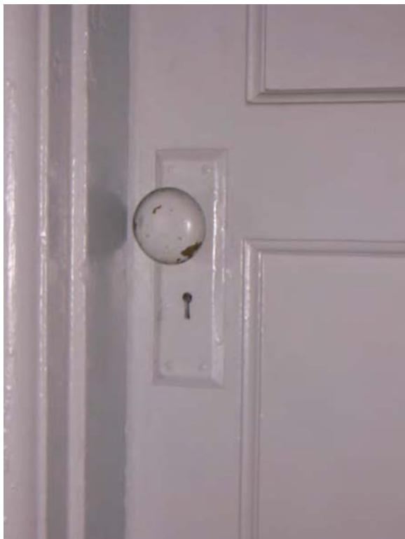
Building 114 – A good example of historic hardware on a wood panel interior door. If hardware needs to be replaced it should replicate the original.
