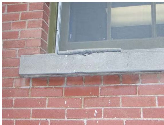
Building 114 – Determine a patching material that is chemically and visually compatible with the building and existing material.
