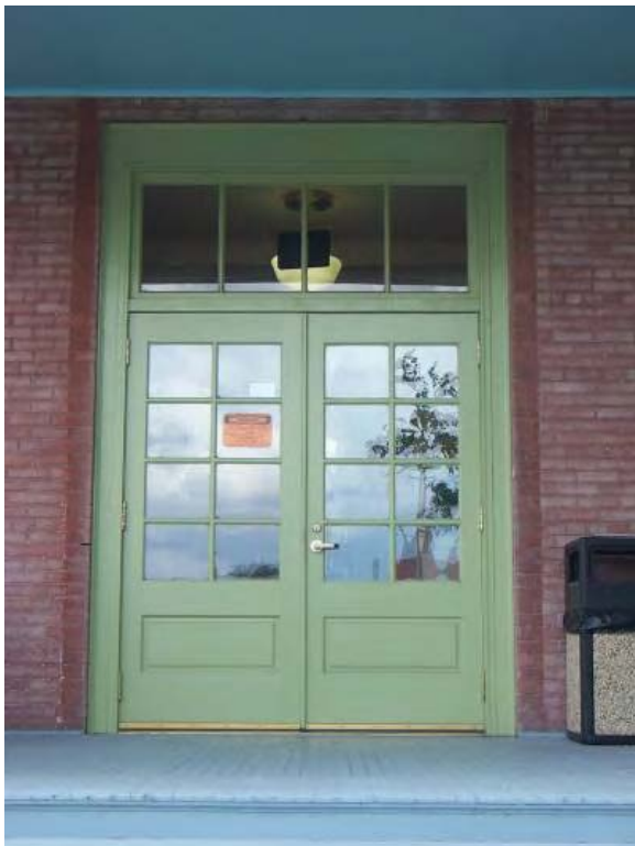
Building 4 – These are appropriate wood doors, wood transom, and door frame replacement types for this building.
