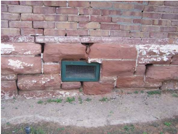
Building 128 – Inspect key areas of the building where sandstone could be located, like the foundation. Examine the overall condition of the sandstone and mortar joints.
