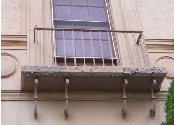
Building 504 – Check for chips in the coating surface and peeling of paint. Here the paint peeling on the concrete balcony may be caused by standing water. Look at the connection between the metal and the concrete.
