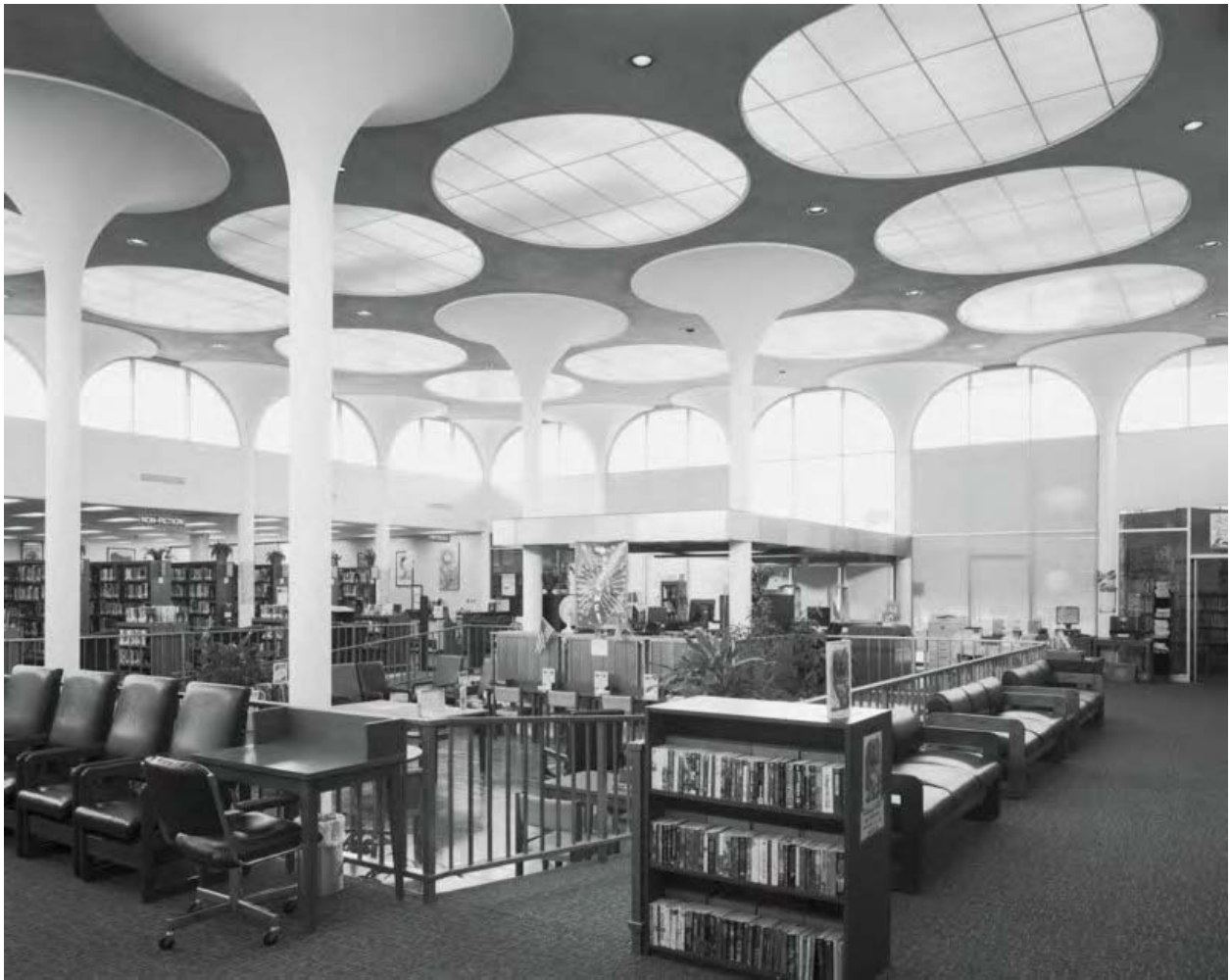
Photo 15 – interior general view from southeast corner, view to southwest.
