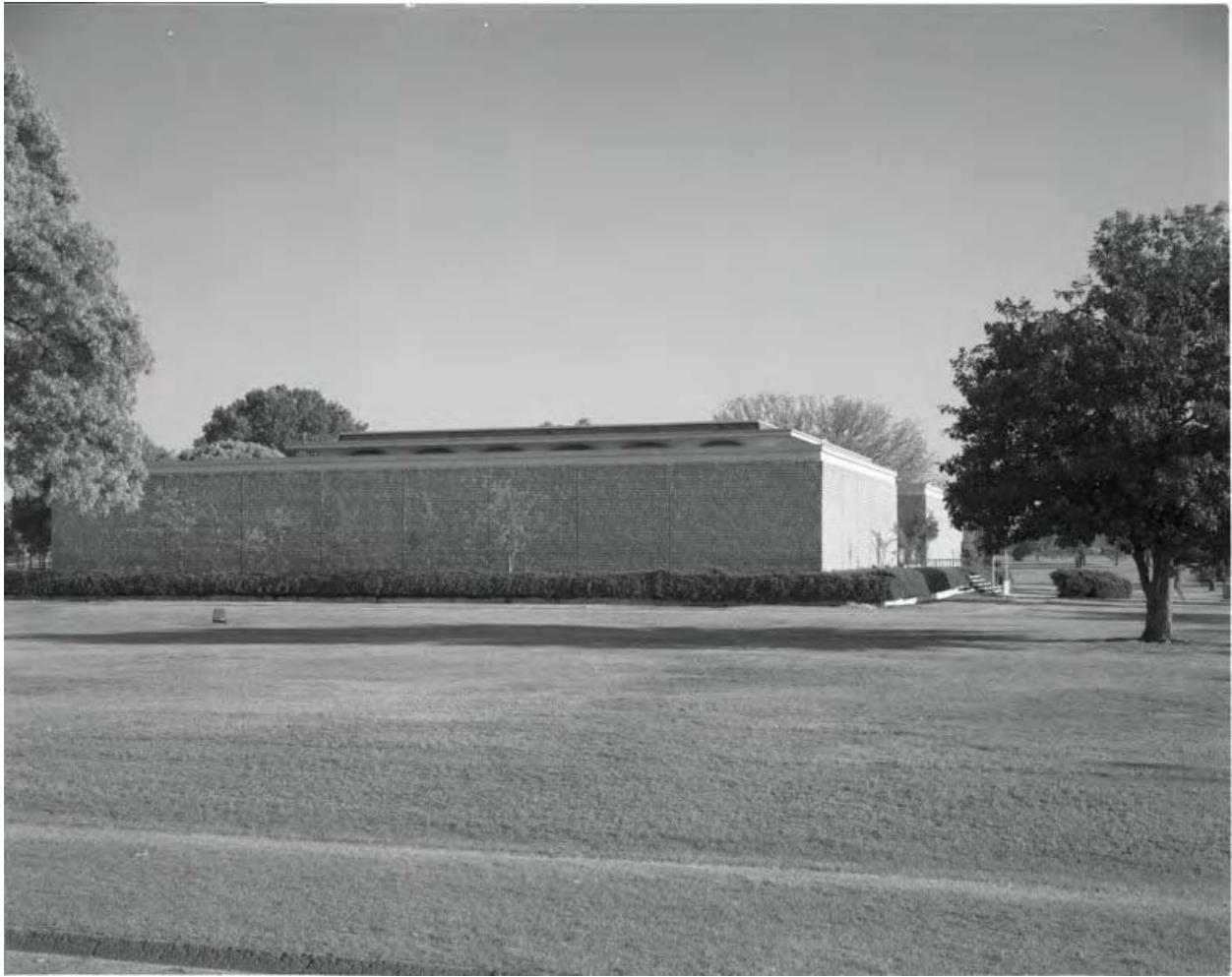
Photo 6 – exterior general view south side and west facade right, view to south.
