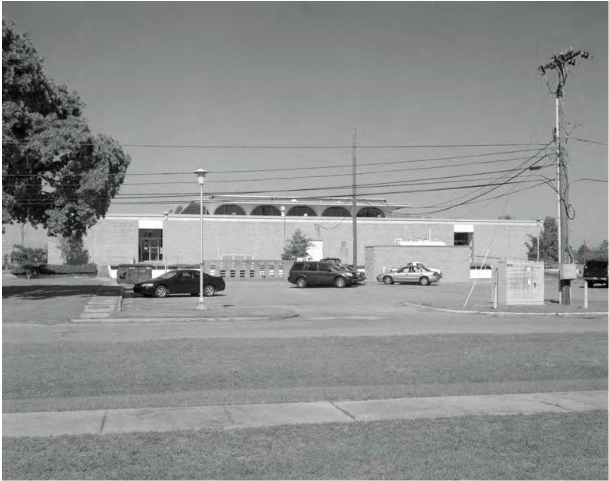
Photo 7 – exterior general view east elevation with loading dock, note clerestory and arches above, view to west.
