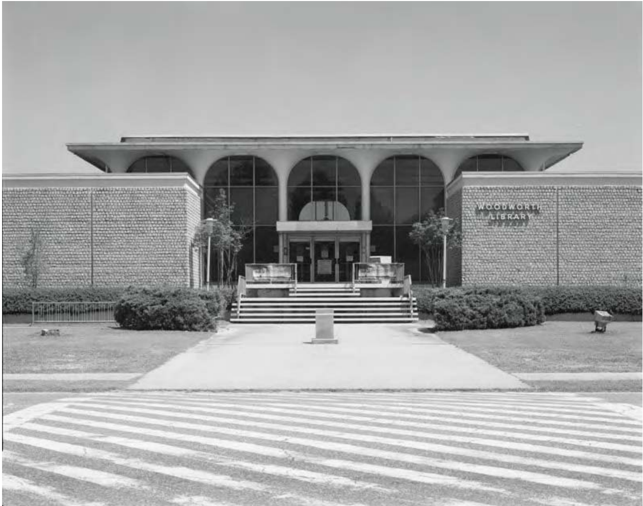
Photo 2 – exterior detail of center west facade and main entry, view to east.
