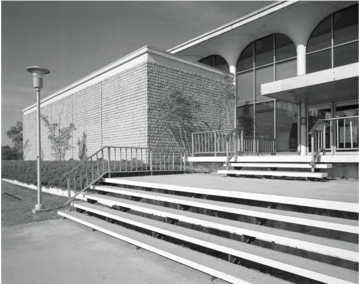
Photo 5 – exterior detail, main central entry area with stairs showing ashlar granite panels northeast module projecting to west, view to northeast.
