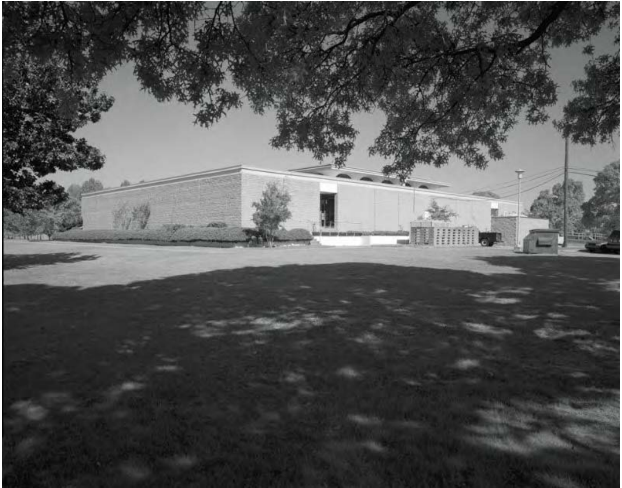
Photo 10 – exterior general oblique view south and east elevations, view to northwest.
