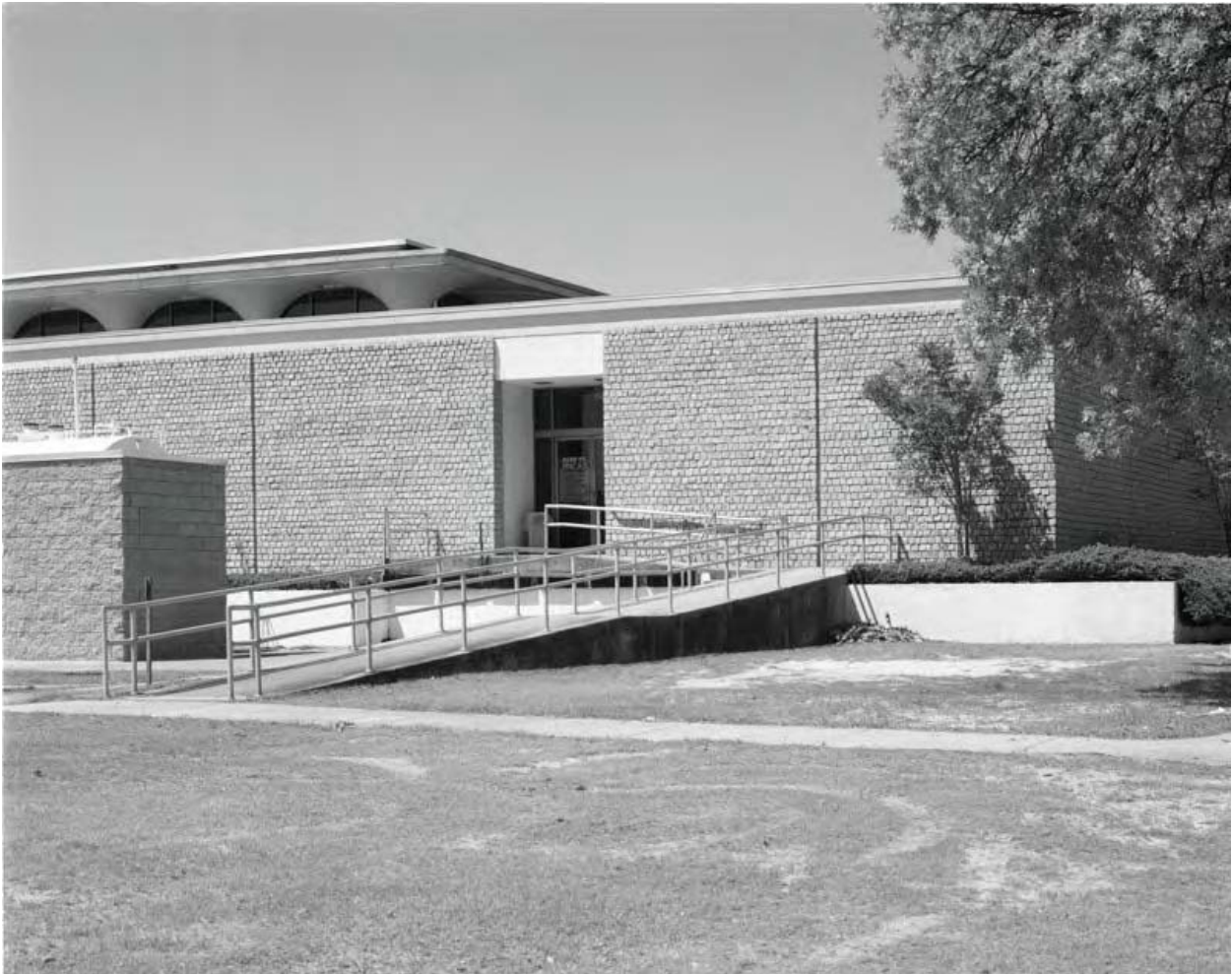
Photo 8 – exterior detail east side, north end, with ADA ramp and employee/service entrance, view to southwest.
