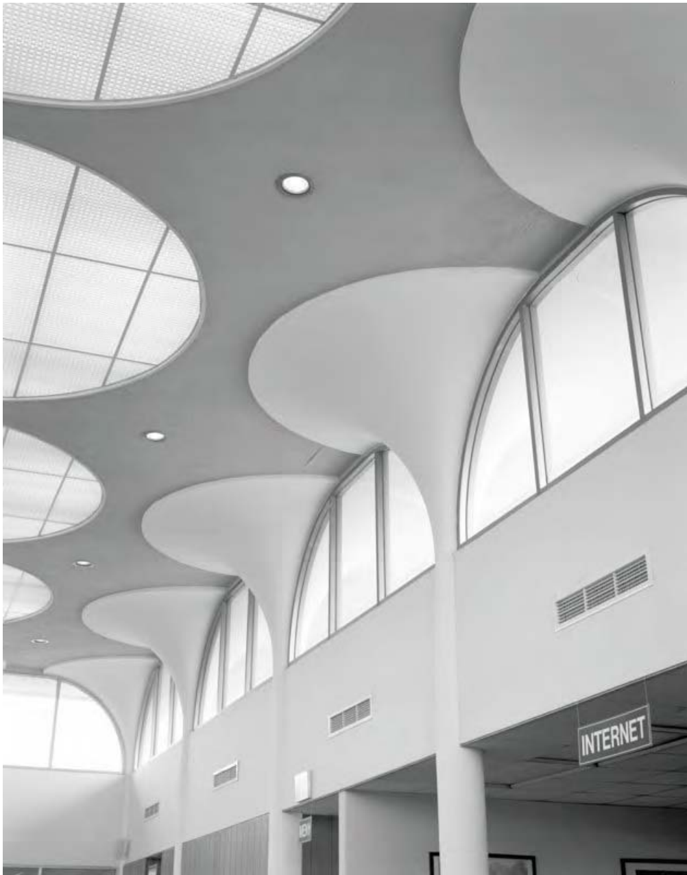
Photo 19 – interior detail, column tops at north side of clerestory section, forming arches for glazing panels, view up and to northwest.
