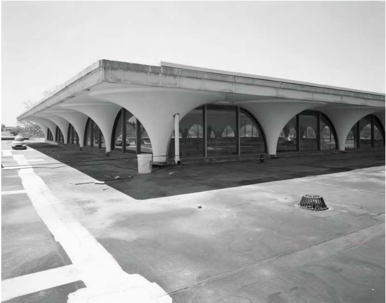
Photo 11 – exterior detail on roof showing tops of “mushroom” capitals forming clerestory, view to southwest.
