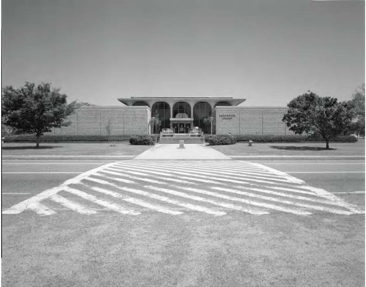
Photo 1 – exterior general view of west main façade, view to east.
