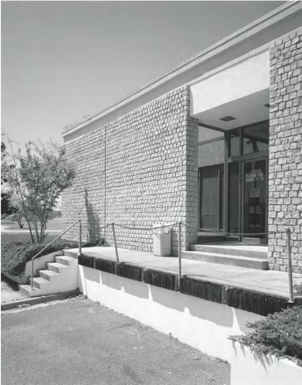
Photo 9 – exterior detail, loading dock at south end of east elevation, showing stairs and recessed entry, view to southwest.
