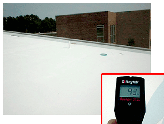
Figure 6. After installation of a cool roof, there was a dramatic decrease in roof surface temperature.
