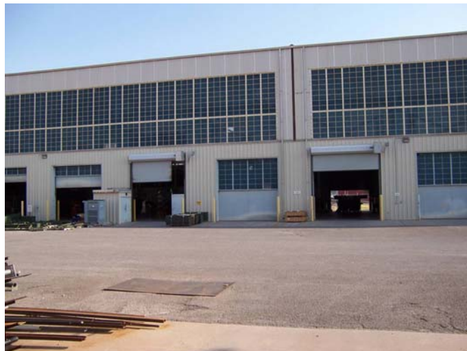
Figure 7. Windows in Maintenance Shop, Bldg. 2588.
