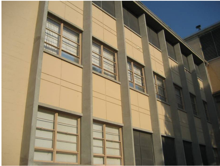
Figure 12. Single pane windows in Bldg. 2.
