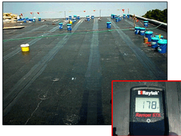
Figure 5. Before installation of a cool roof, a thermometer at the original roof surface reads 178 °F on a hot summer afternoon.
