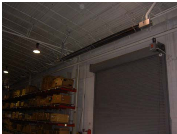
Figure 29. Interior of Medical Warehouse (Bldg. 11156) is very dark, even with artificial lighting.
