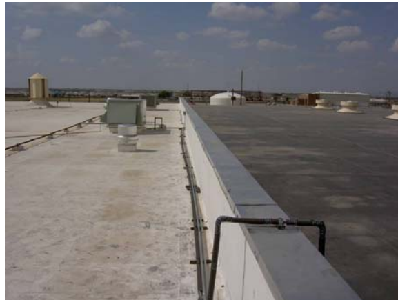
Figure 4. White and black sections of roof of Medical Warehouse, Bldg. 11156.
