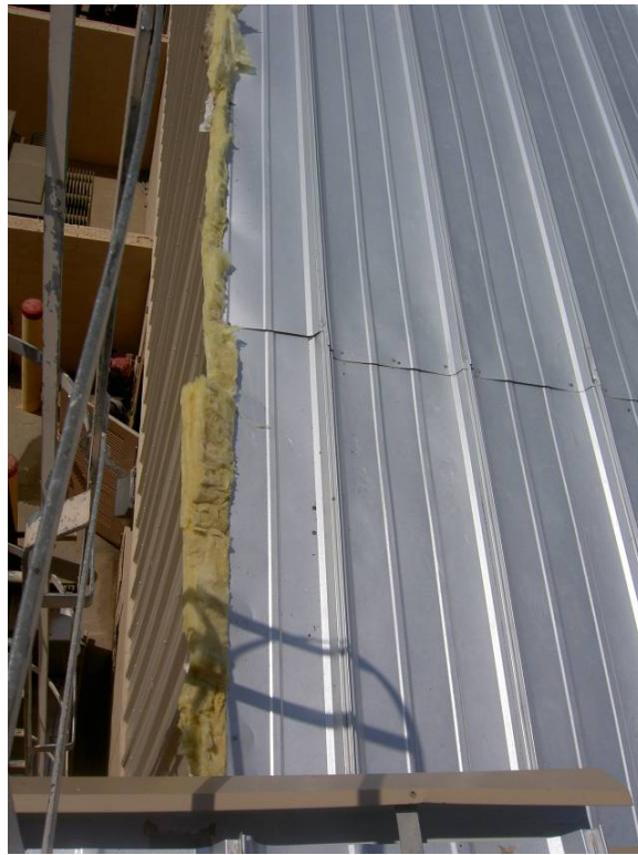
Figure 3. “Un-cool” roof installed on Bldg. 2629.
