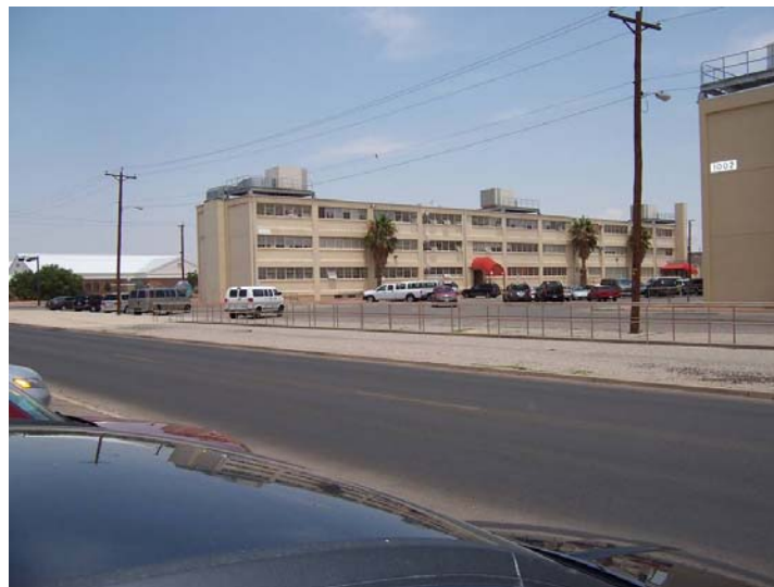
Figure 9. Barracks building with old windows.
