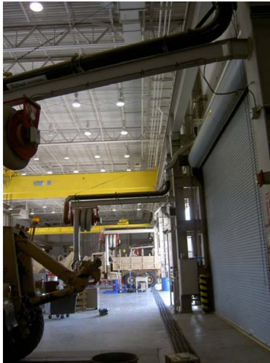
Figure 31. Electric lights in use when natural daylighting is available.
