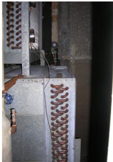
Figure A-6. Hot and Chilled Water Decks
